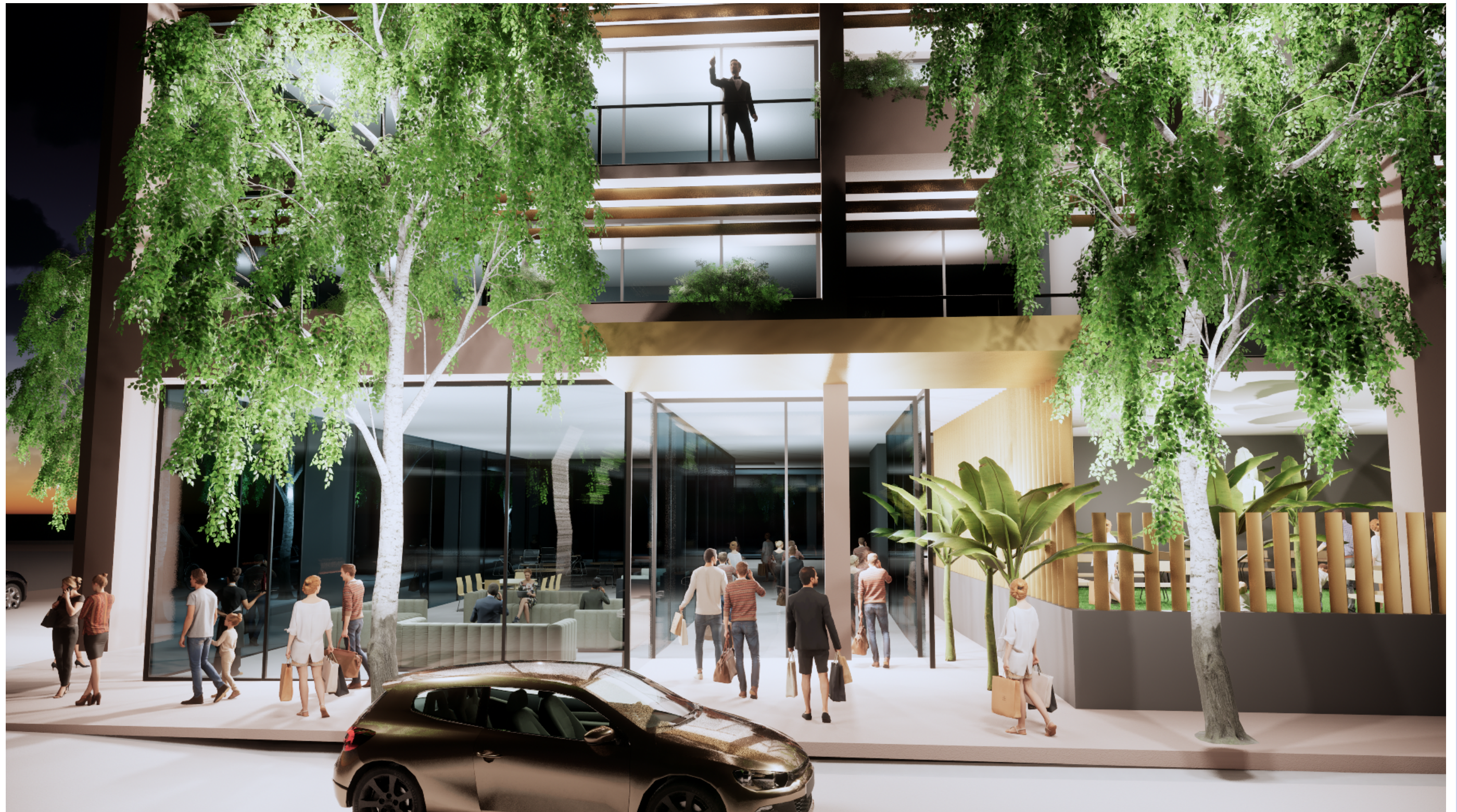
ARTISTS IMPRESSION OF THE MAIN PEDESTRIAN ENTRY TO THE GROUND FLOOR FOYER OFF LOFTUS LANE
