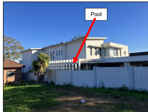
Figure 14: 85 Newton Road, as viewed from the rear yard of the subject site
