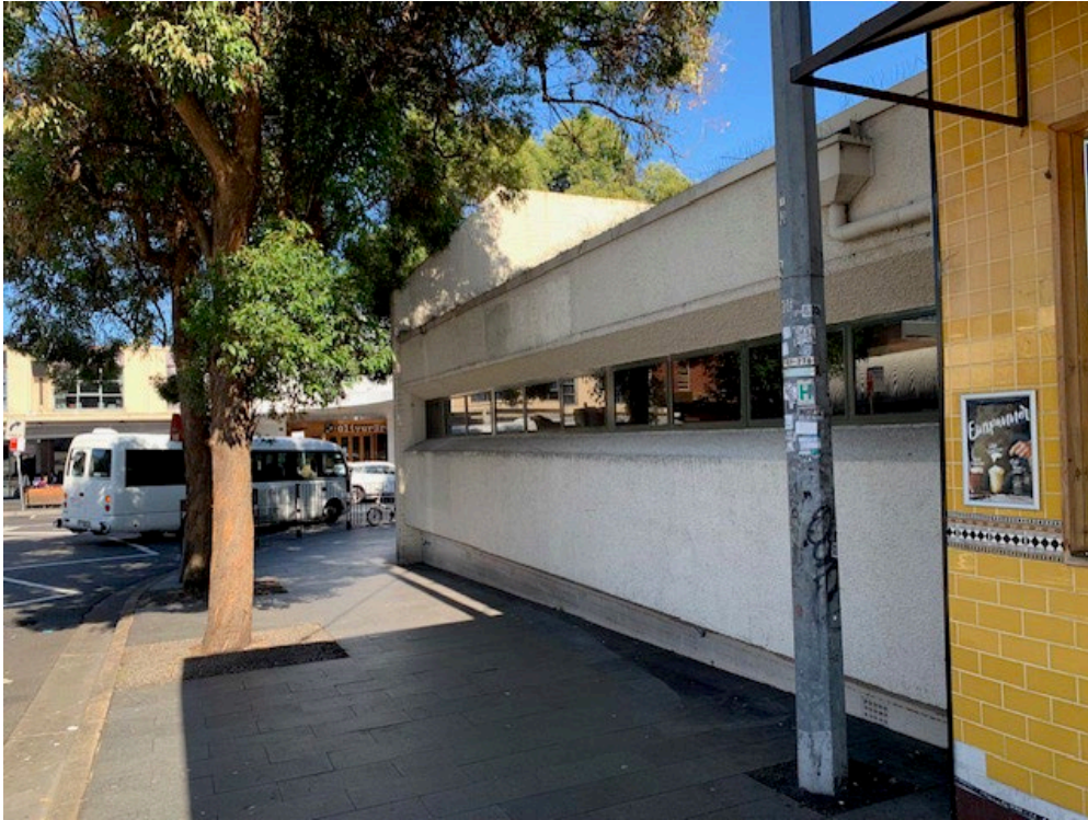
Figure 9: Existing vacant commercial building facing southwest towards Strathfield Plaza
