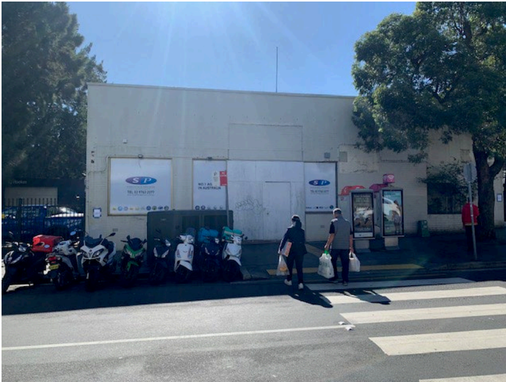
Figure 7: Existing vacant commercial building from Churchill Avenue
