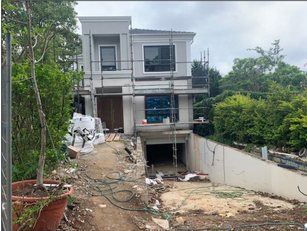
Figure 12: Dwelling at 175 Albert Road nearing completion
