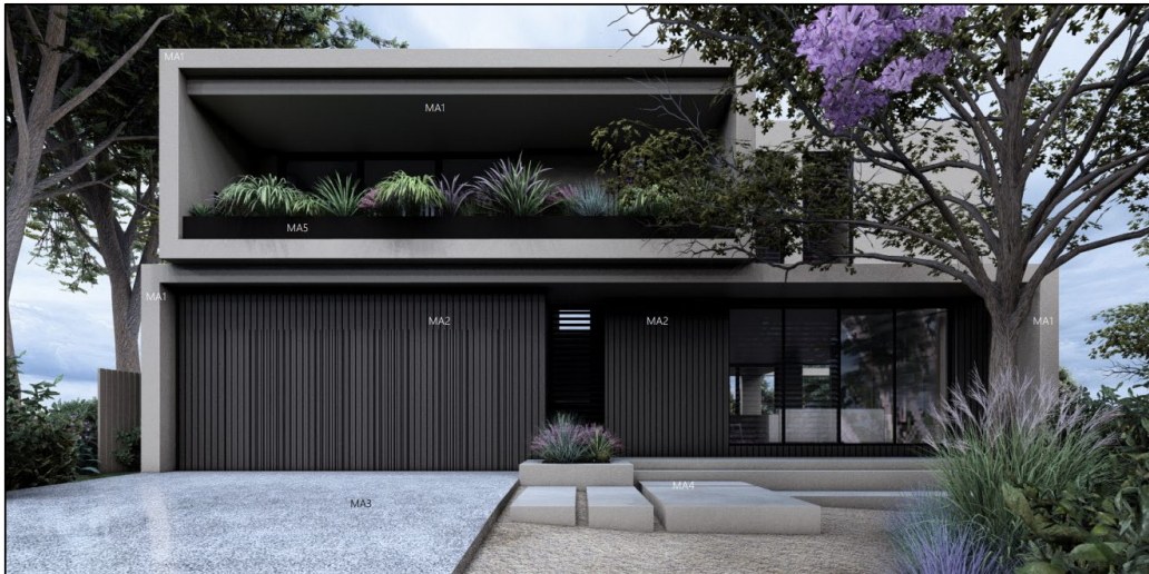
Figure 6: Front Façade Montage
