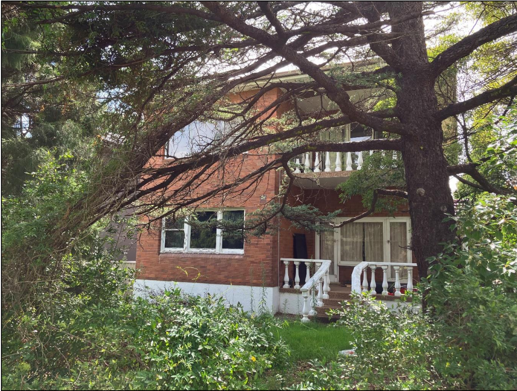
Figure 14: Front façade of the existing dwelling to Pemberton Street
