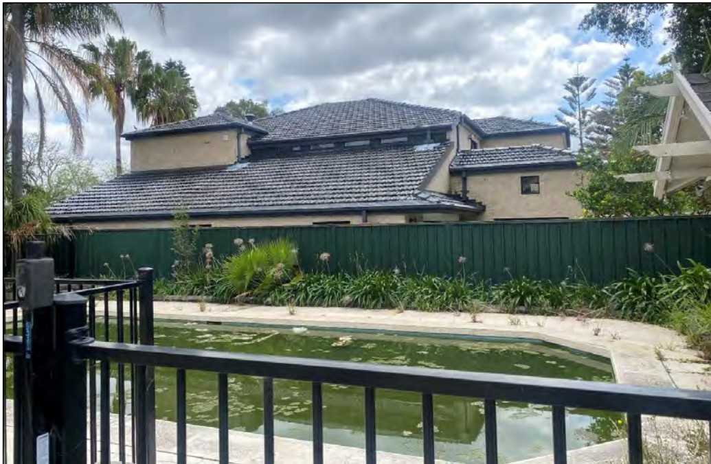
Figure 26: Rear yard of dwelling facing north toward site's northern side boundary.
