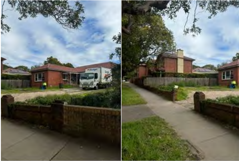
Figure 2: Subject site as viewed from Homebush Road.
