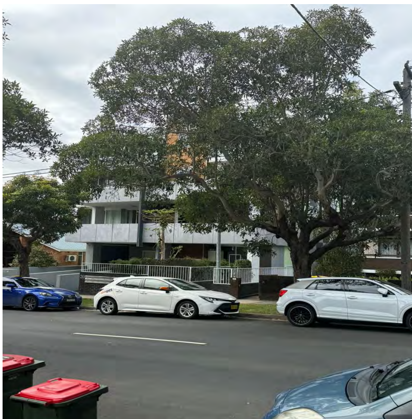
Figure 6: Neighbouring 4 storey apartment building on the eastern side of Homebush Road.
