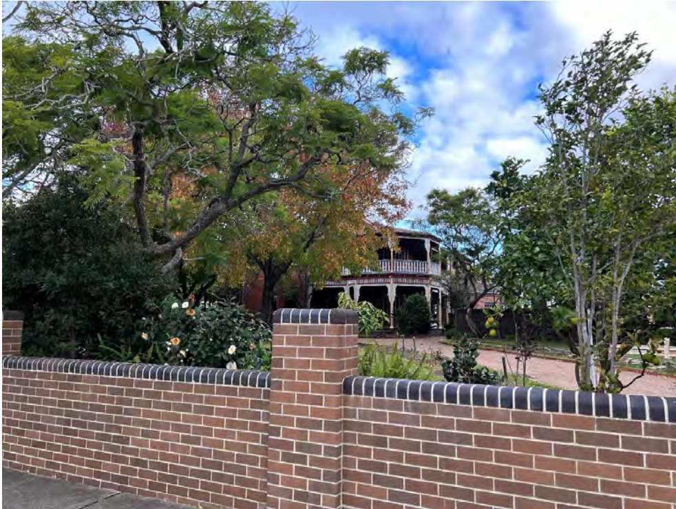
Figure 17: Existing dwelling house at the subject site as viewed from Llandilo Avenue
