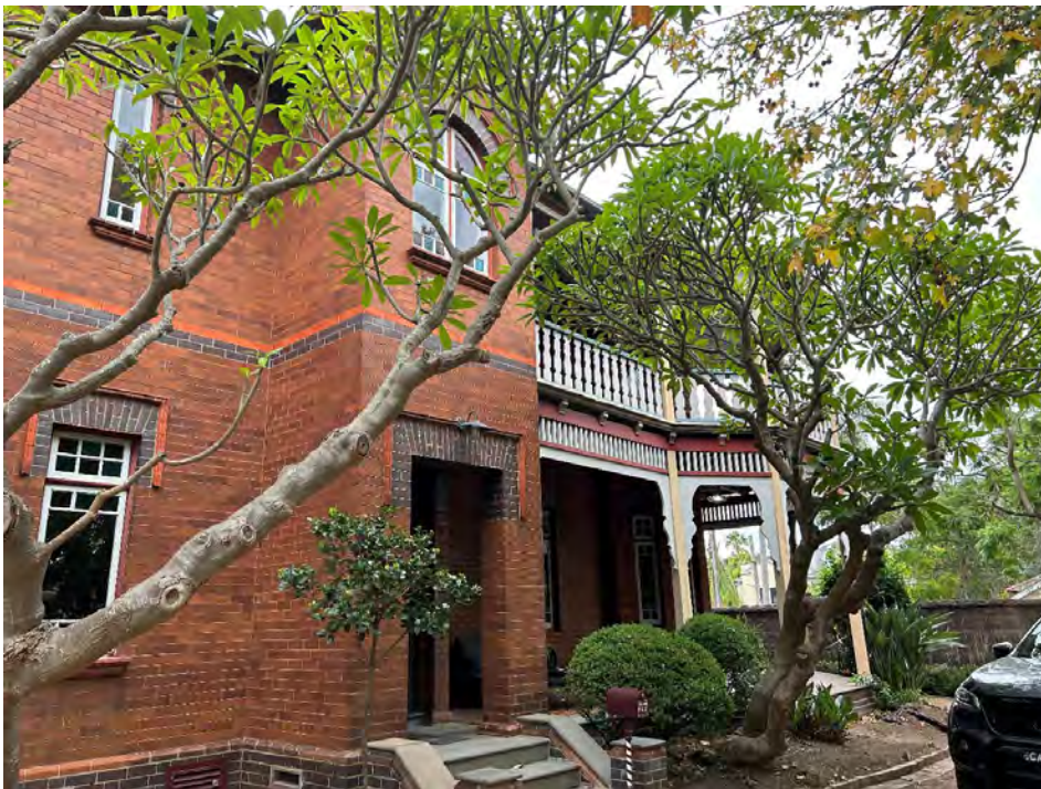
Figure 25: Existing front entry and northern facade
