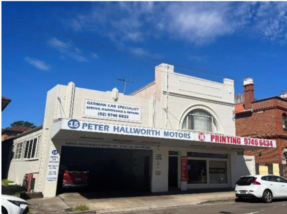
Figure 4: Adjoining commercial building to the east at 15-16 The Crescent.
