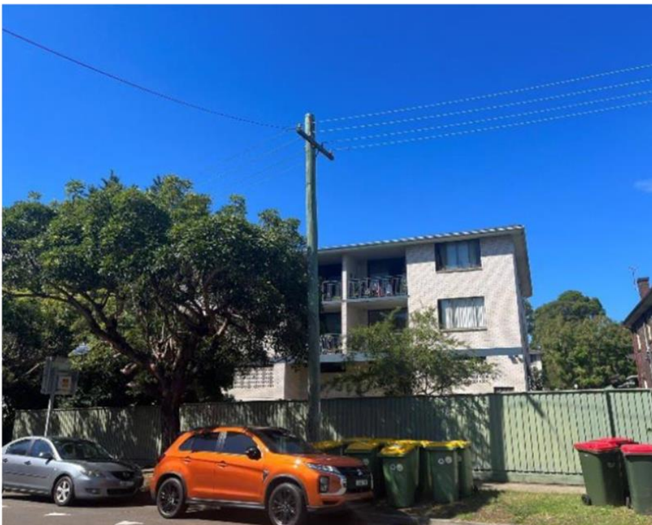
Figure 3: Adjoining residential flat building to the east at 7-9 Burlington Road.
