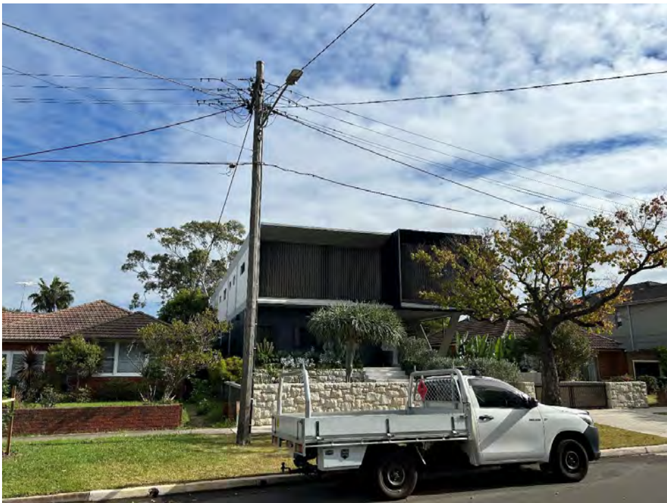
Figure 17: Existing dwelling at the site
