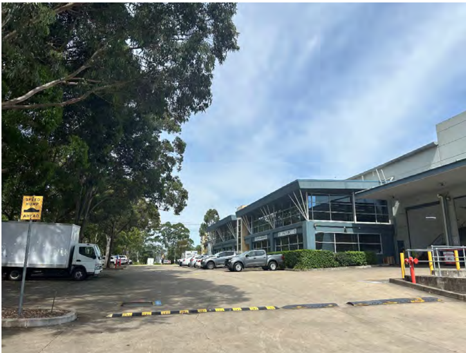
Figure 23: View from exit point onto the internal private road, looking south back towards Arthur Street
