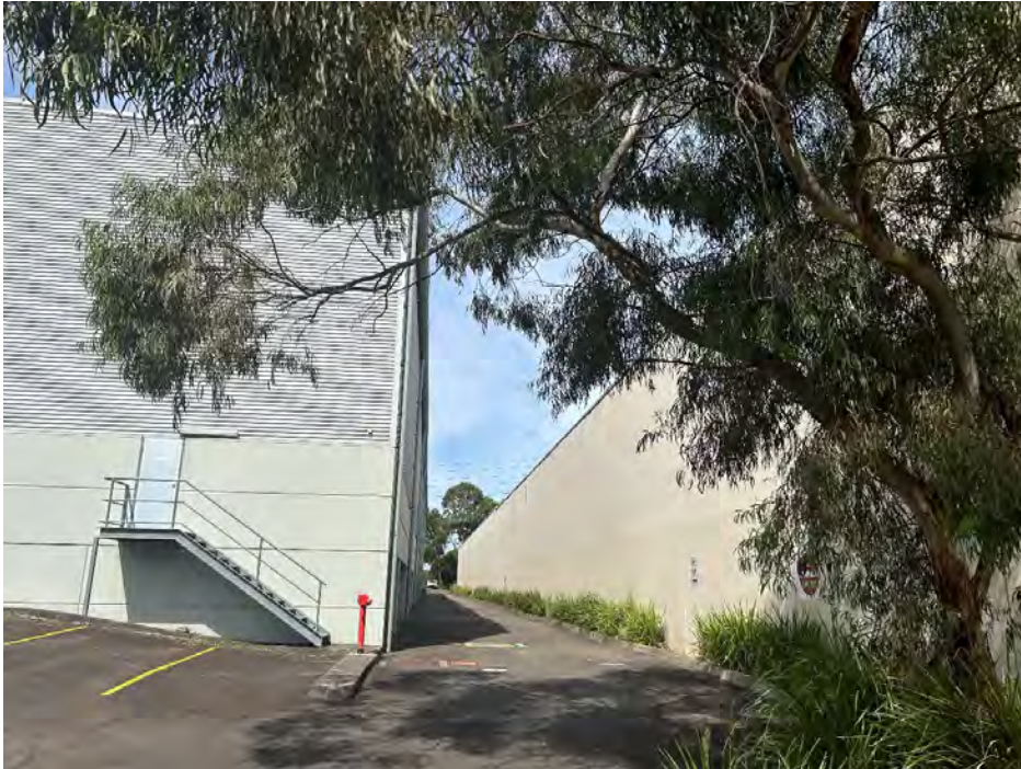
Figure 20: View of the western end of the northern façade of the warehouse to be extended. Site access runs along the western boundary with undercroft parking. The tree on the right is proposed for removal.
