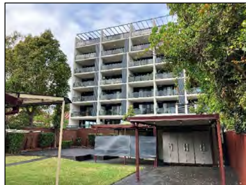
Figure 19: The rear of 10 Kanoona Avenue, viewed towards the south east
