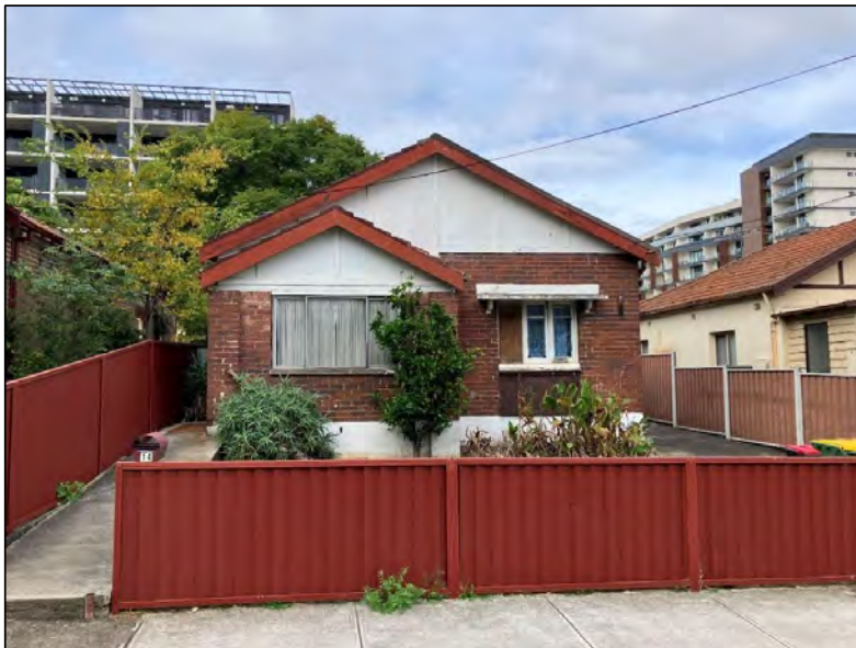
Figure 23: Adjoining development at 14 Kanoona Avenue, as viewed from the street
