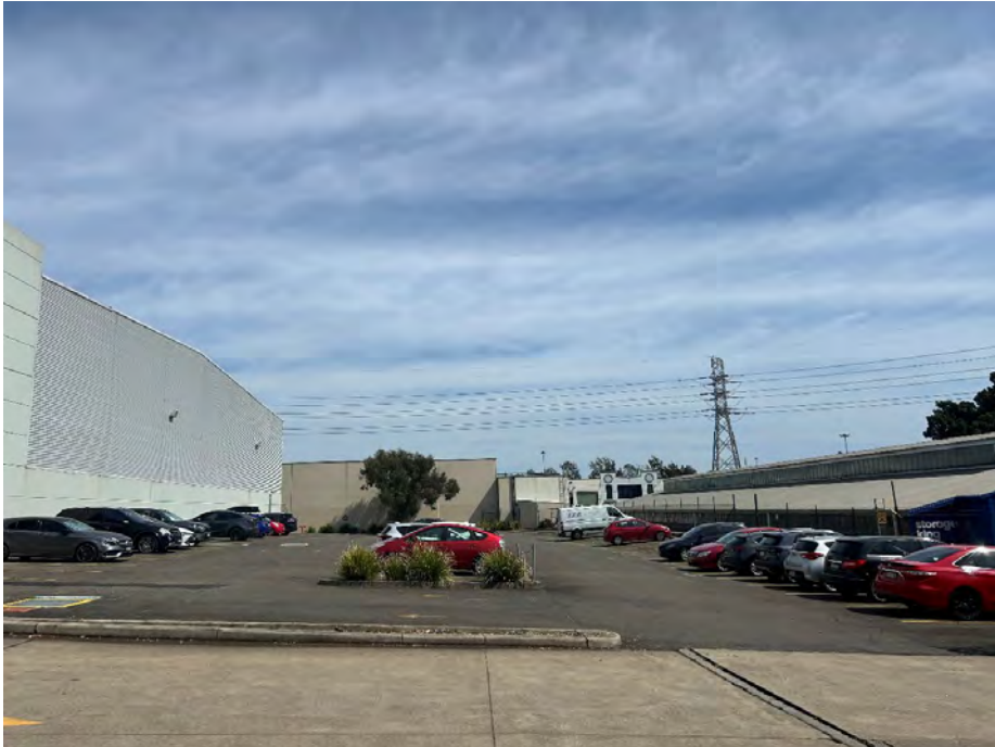
Figure 18: View of the car park to be demolished and developed, looking west
