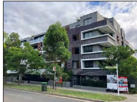
Figure 27: Residential flat building on the other side of the road at 1-9 Kanoona Avenue
