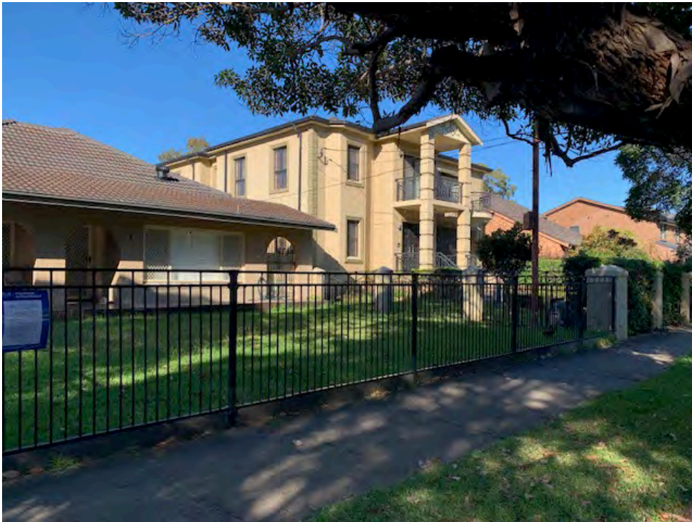
Figure 18: 100 Beresford Road, as viewed from the street
