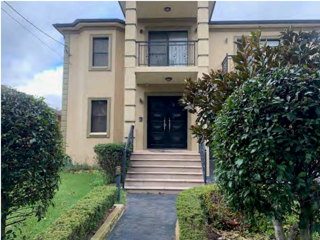
Figure 24: 100 Beresford Road, ground floor protrudes substantially out of natural ground level.
