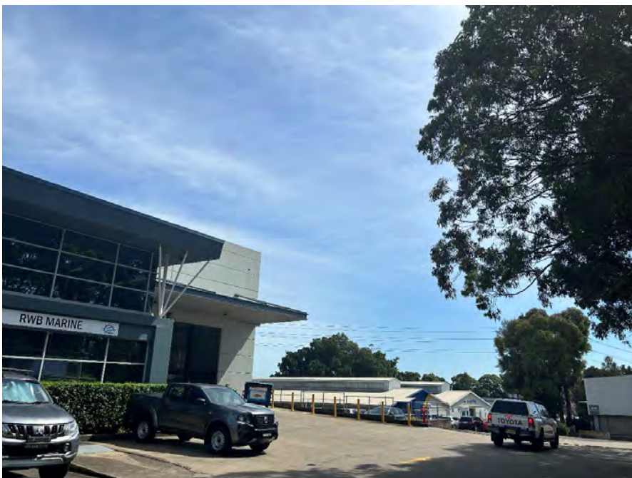
Figure 17: Looking north-west at the development site. The extension will be attached to the existing warehouse with the pale green façade and awning
