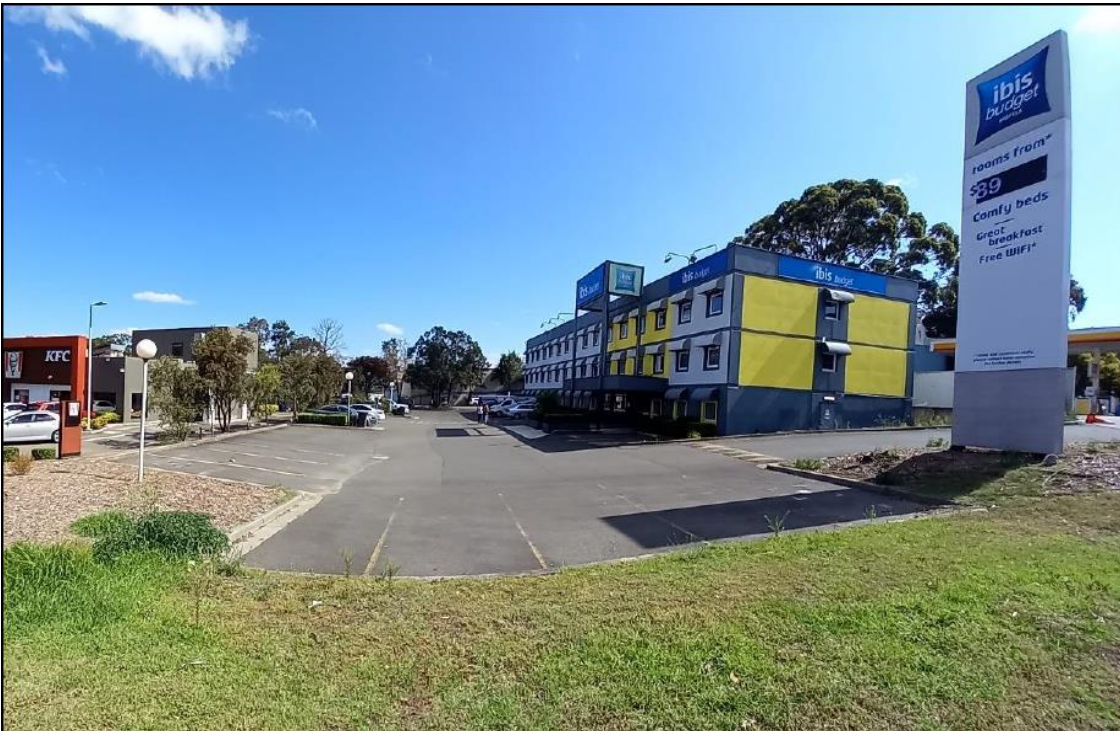
Figure 14: Subject site existing hotel development
