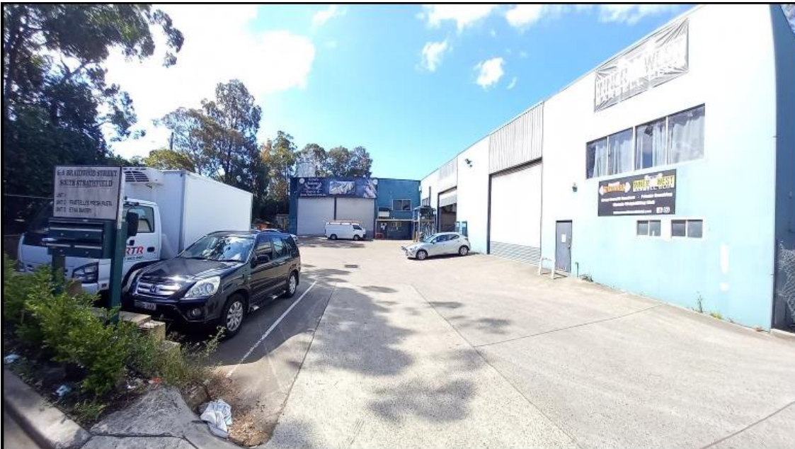
Figure 18: Existing warehouse development at 6 Braidwood Street
