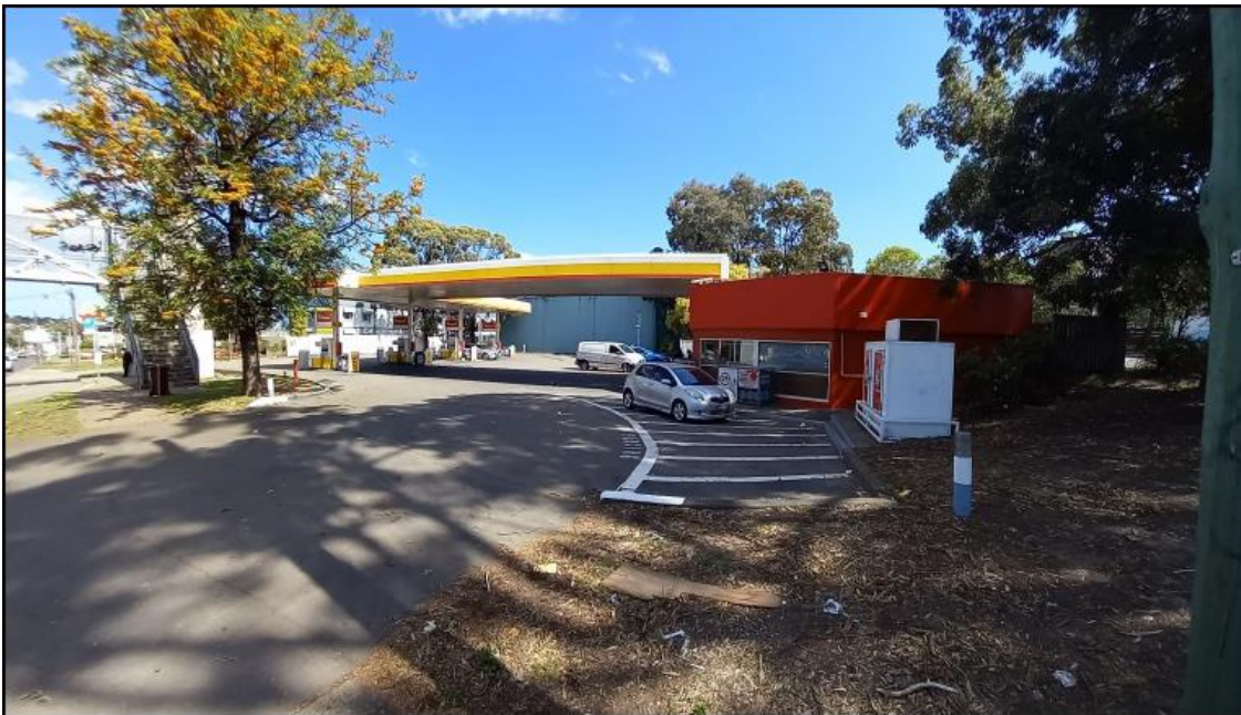
Figure 17: Existing service station at 630-634 Liverpool Road
