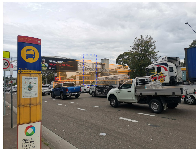
3. VIEW FROM LIVERPOOL ROAD. 48 m from Subject Site
