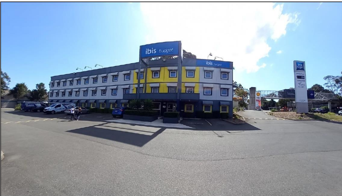
Figure 15: Subject site existing hotel development east elevation
