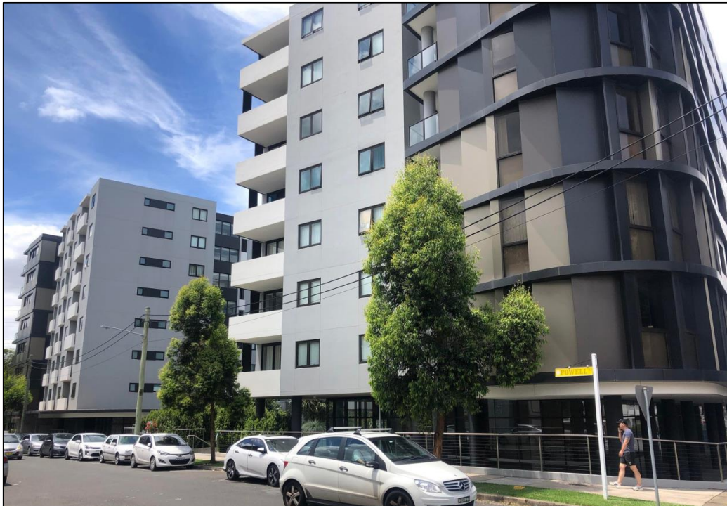
Figure 17: Two existing 8 storey mixed use flat buildings east of the site at 17-35 Powell Street.
