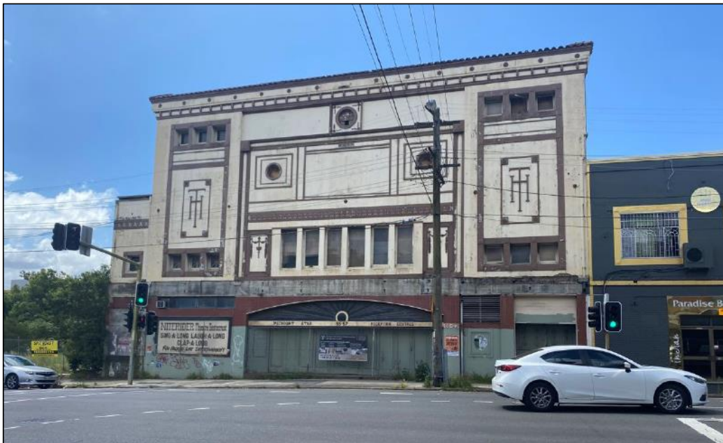
Figure 14: Homebush Theatre Site fronting Parramatta Road.
