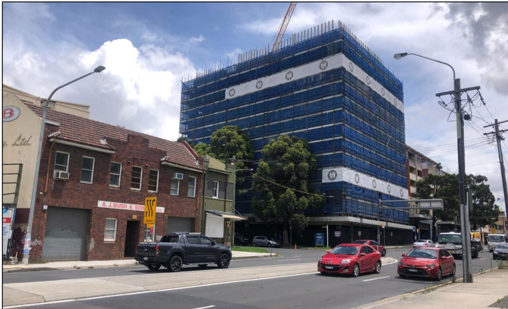
Figure 21: Streetscape comprising some original structures and new high rise development.
