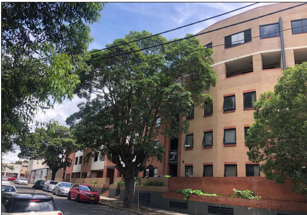
Figure 16: Northern adjoining five storey residential flat building at 2-10 Powell Street.
