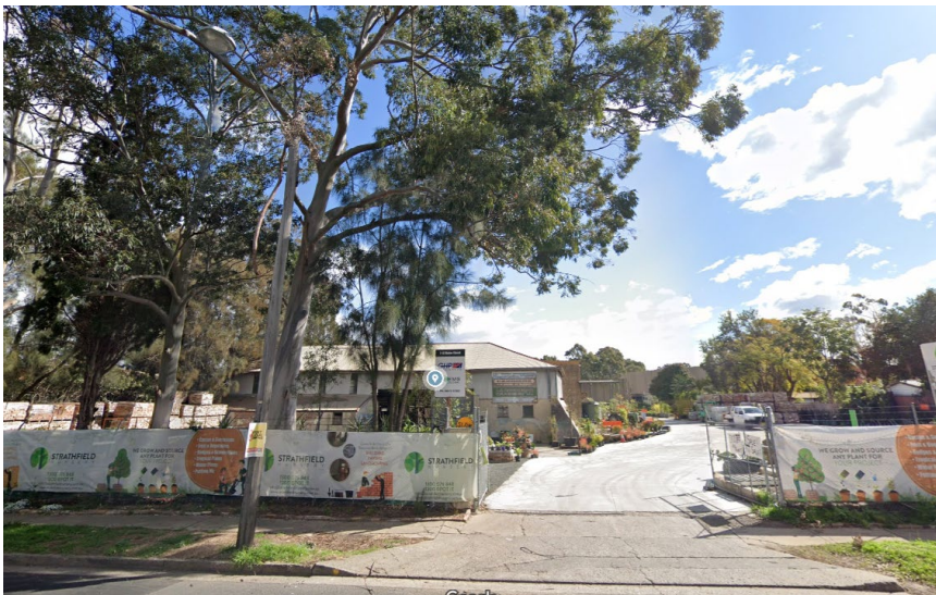
Figure 22 – Northernmost driveway crossover
