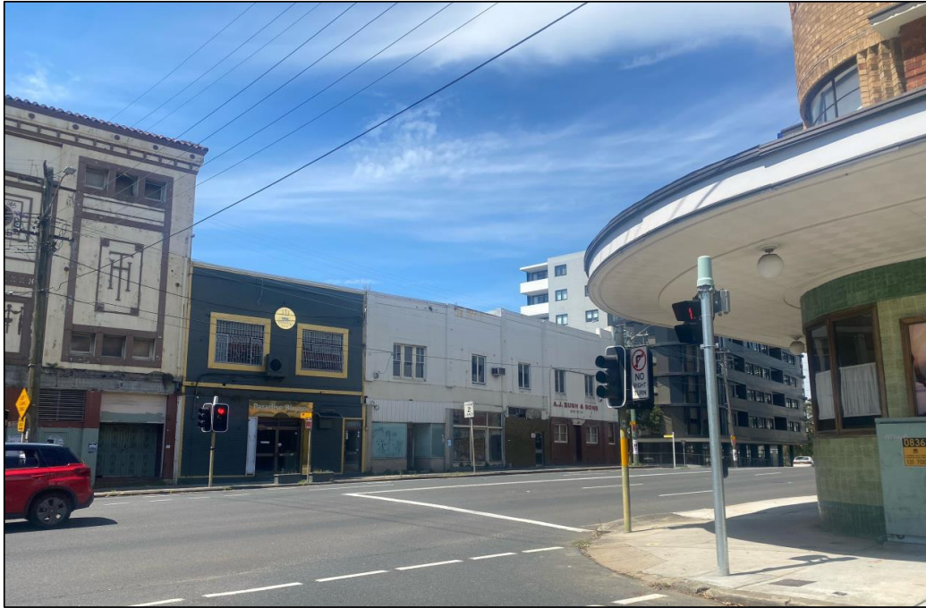
Figure 13: Subject site as viewed from Parramatta Road featuring three attached, two storey retail premises with a primary frontage to Parramatta Road (51 – 53 Parramatta Road). Homebush theatre to far left.
