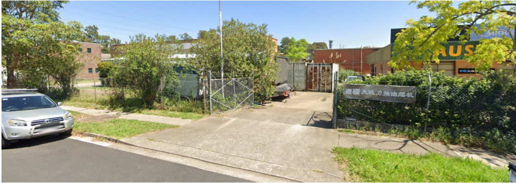
Figure 21 – Southernmost driveway crossover at the site and adjoining industrial development
