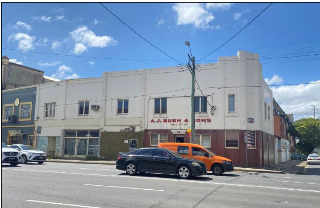
Figure 12: Subject site including AJ Bush & Sons building and commercial tenancies fronting Parramatta Road.
