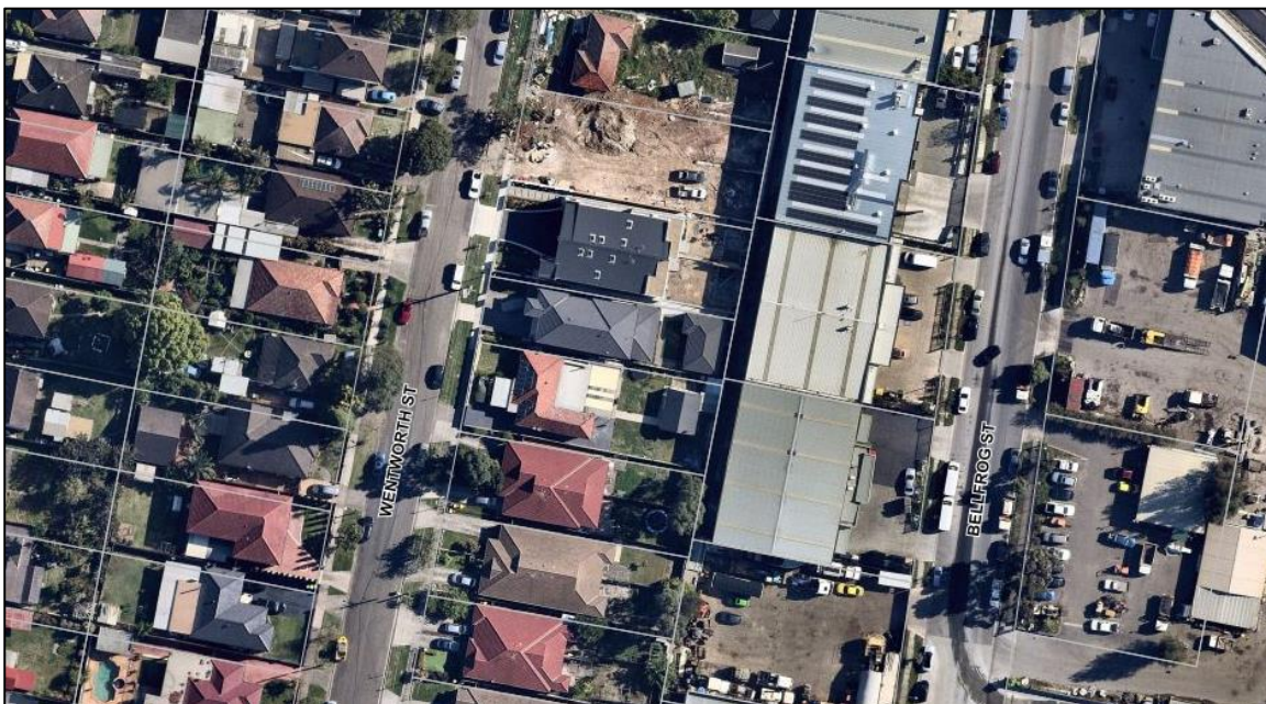
Figure 1: Aerial view of subject site and surrounding context. Subject site outlined in yellow.
