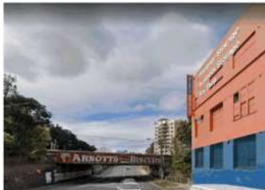
Figure 2 View from Parramatta Road heading east to KSS Homebush site and Railway bridge with Arnotts sign Source: Google Map
