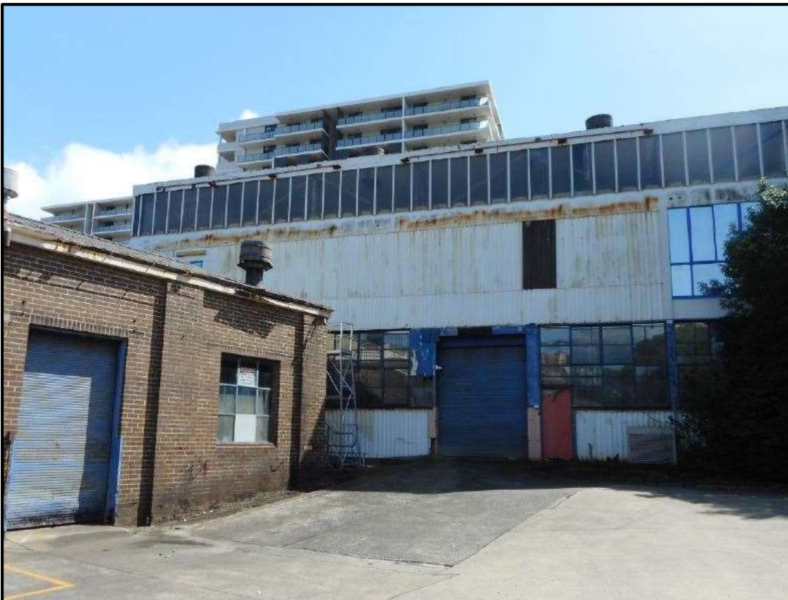
Figure 7: Southern side of southern building.
