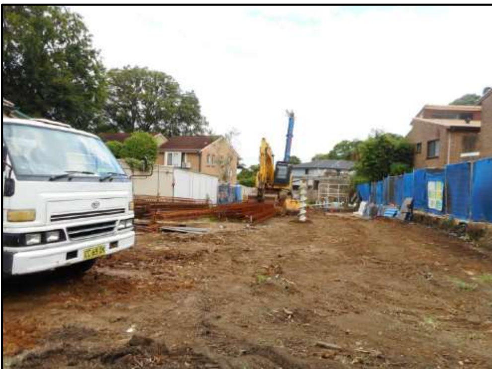
Figure 2: View of site from front boundary – towards northern (rear) boundary.
