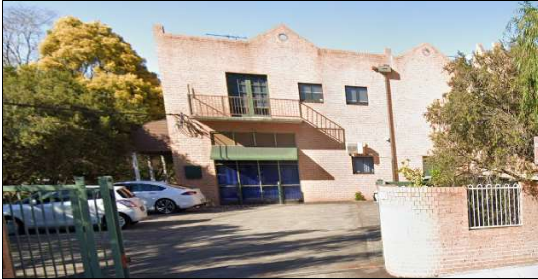
Figure 3: Existing development at 30-32 Pomeroy Street, Homebush
