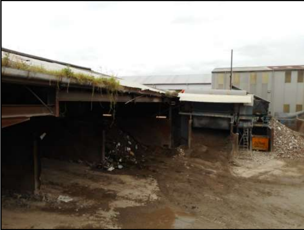
Figure 4. Existing storage bays in western portion of site.
