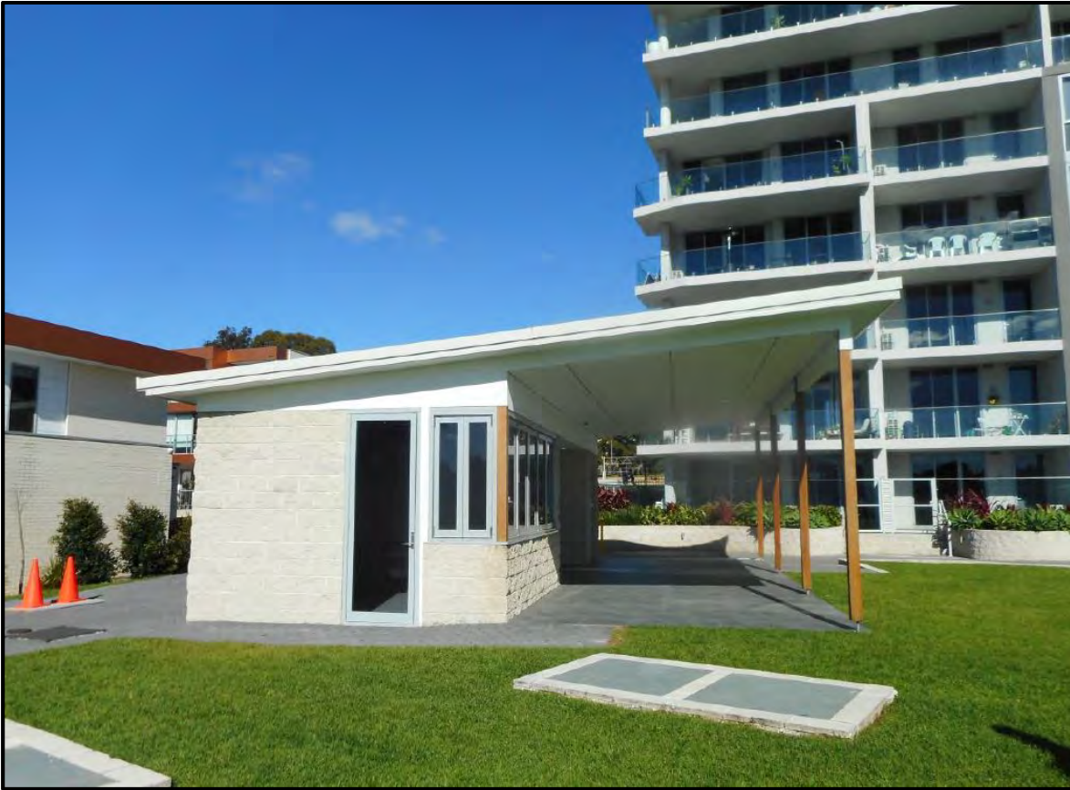
Figure 6: Northern side of kiosk building
