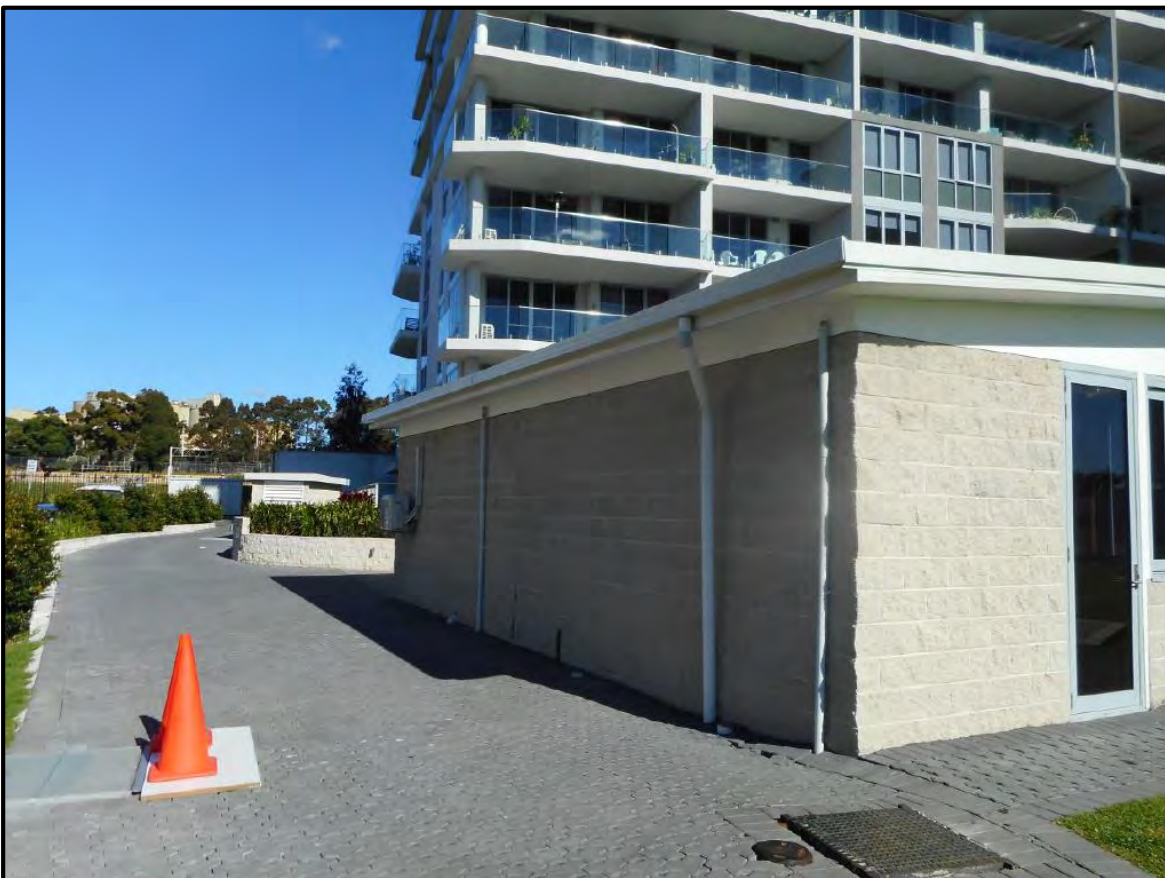
Figure 7: Eastern side of kiosk building
