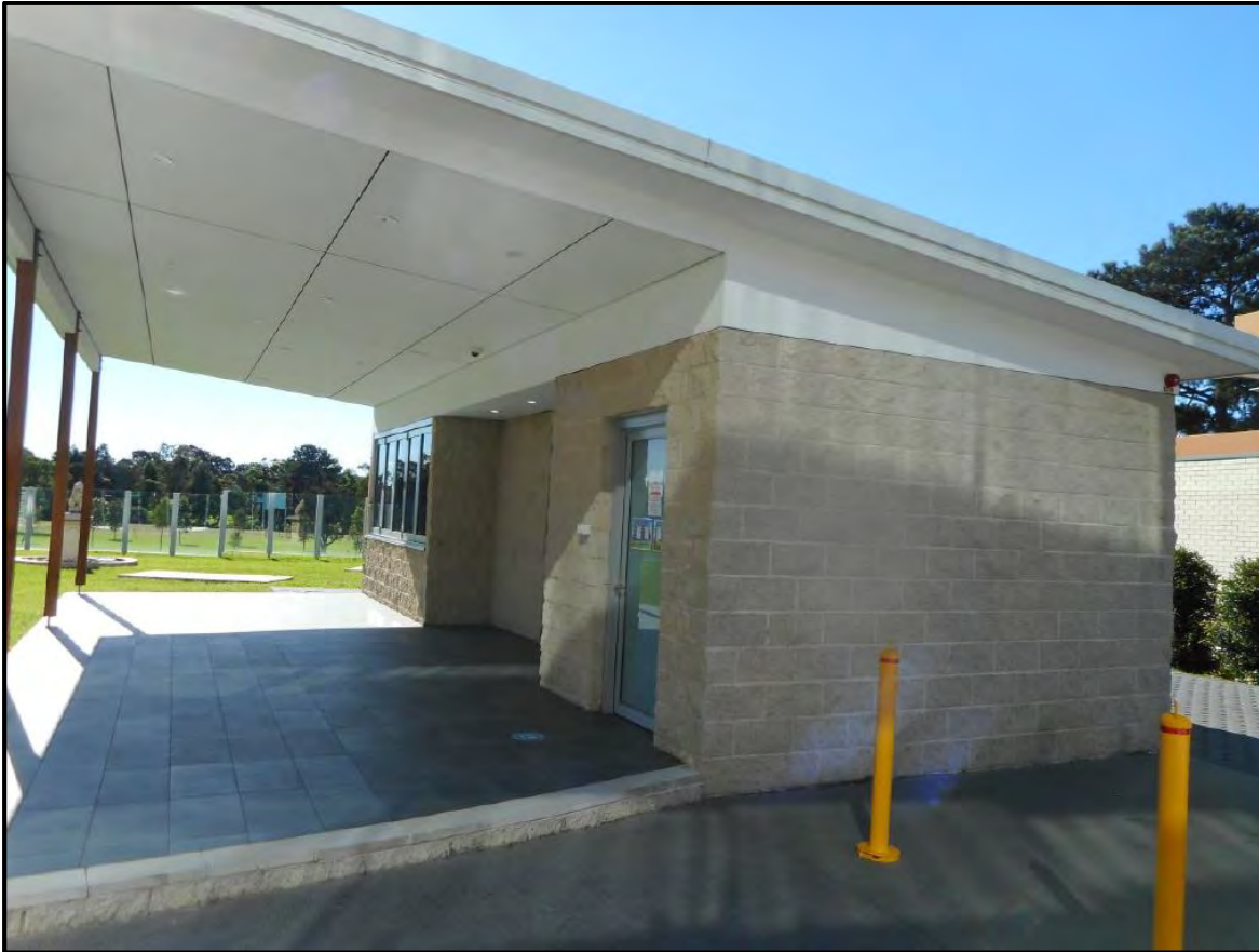
Figure 8: Southern side of kiosk building
