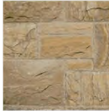
Entry Portico Feature - Sandstone Clad Infill
