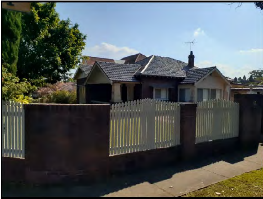
Figure 4: Dwelling at 31 South Street STRATHFIELD
