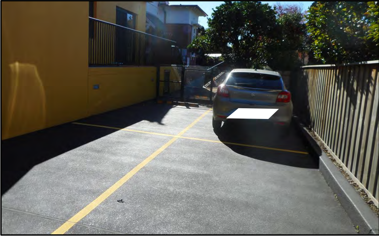
Figure 4: Existing parking spaces for staff – located on the eastern side of the building
