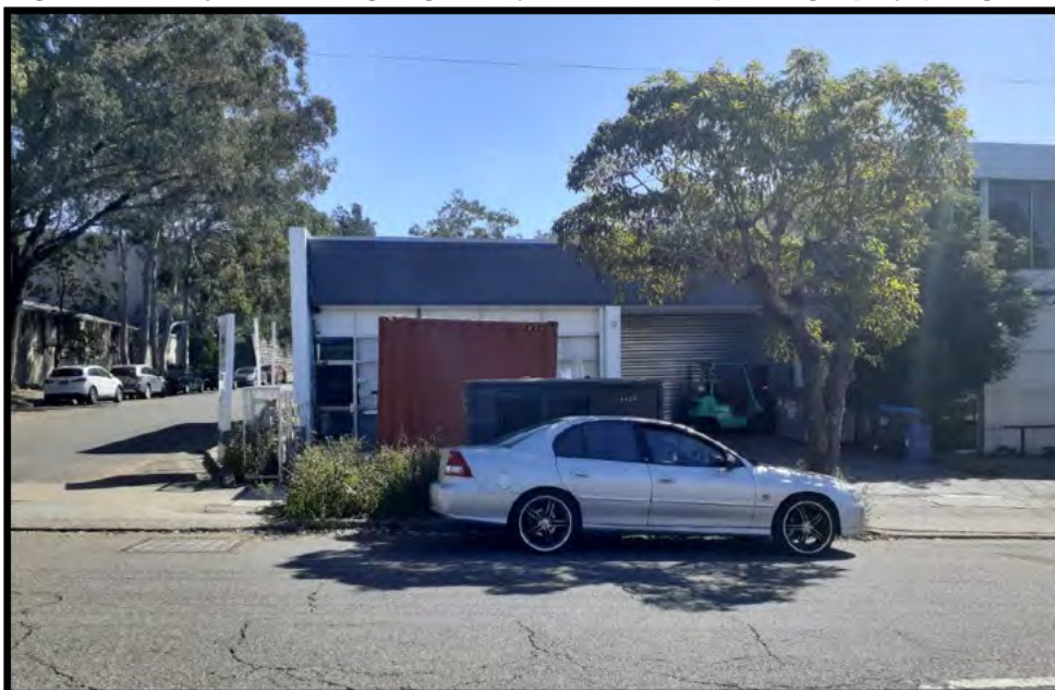
Figure 2: Subject site and existing tree (east elevation)
