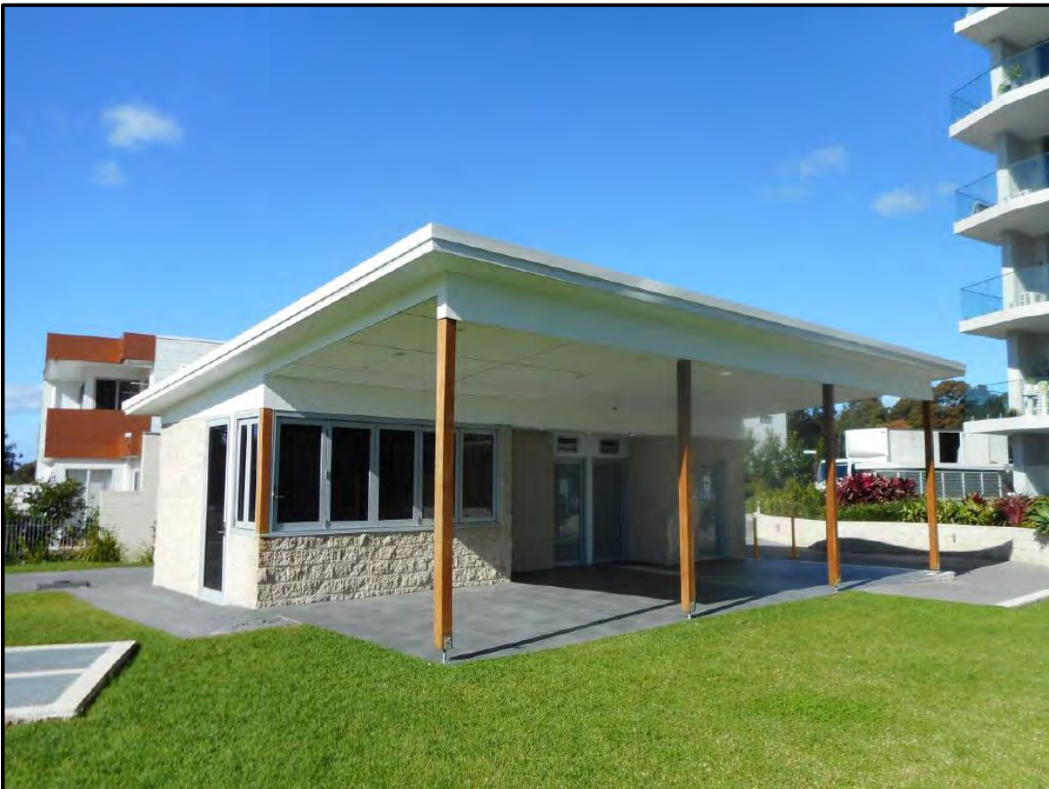
Figure 5: Western side of kiosk building with attached pergola
