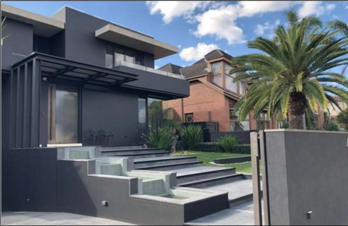
Figure 18: Photo of modern style design at No. 45 Newton Road
