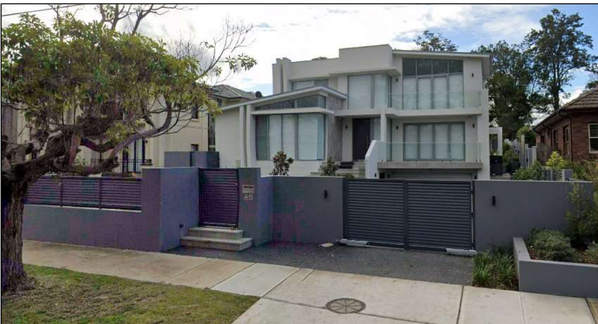
Figure 19: Image of modern style design at No. 85 Newton Road
