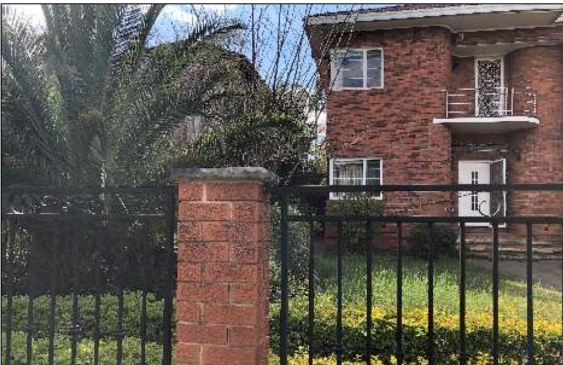
Figure 15: Photo of boundary between No. 43 and No. 41 Newton Road
