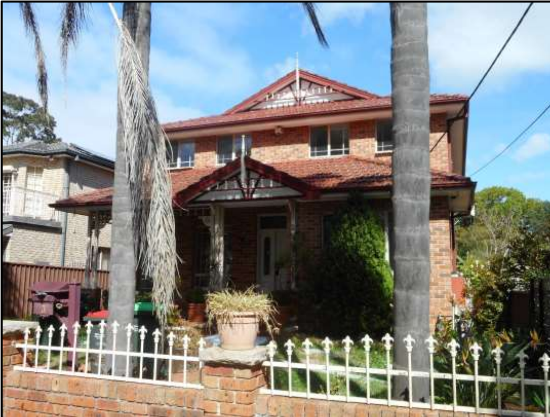
Figure 15. Dwelling house at No. 3 Heyde Avenue
