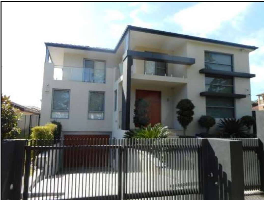
Figure 14. Dwelling house at No. 4 Heyde Avenue
