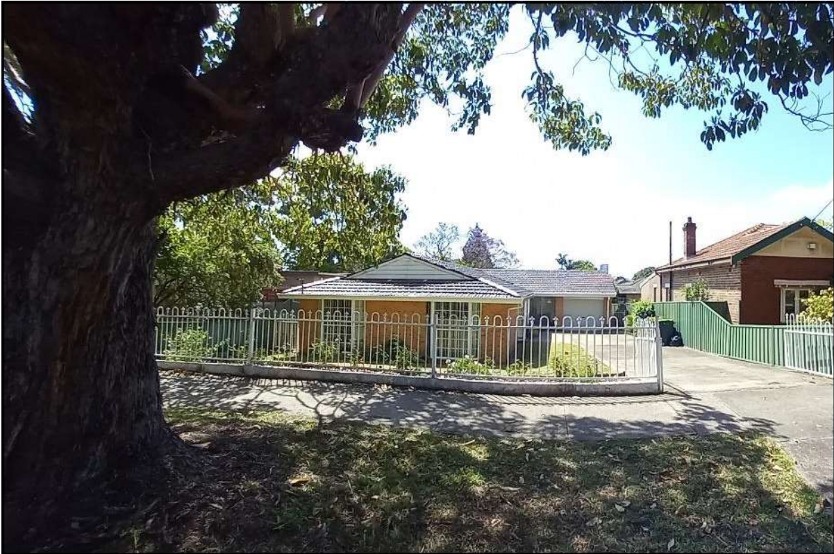
Figure 15: Existing dwelling at 5 Badgery Avenue
