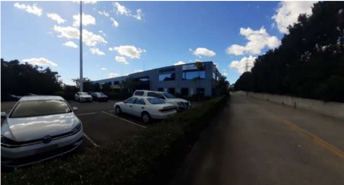
Figure 31: Existing south-west carpark and office building (east-facing)
