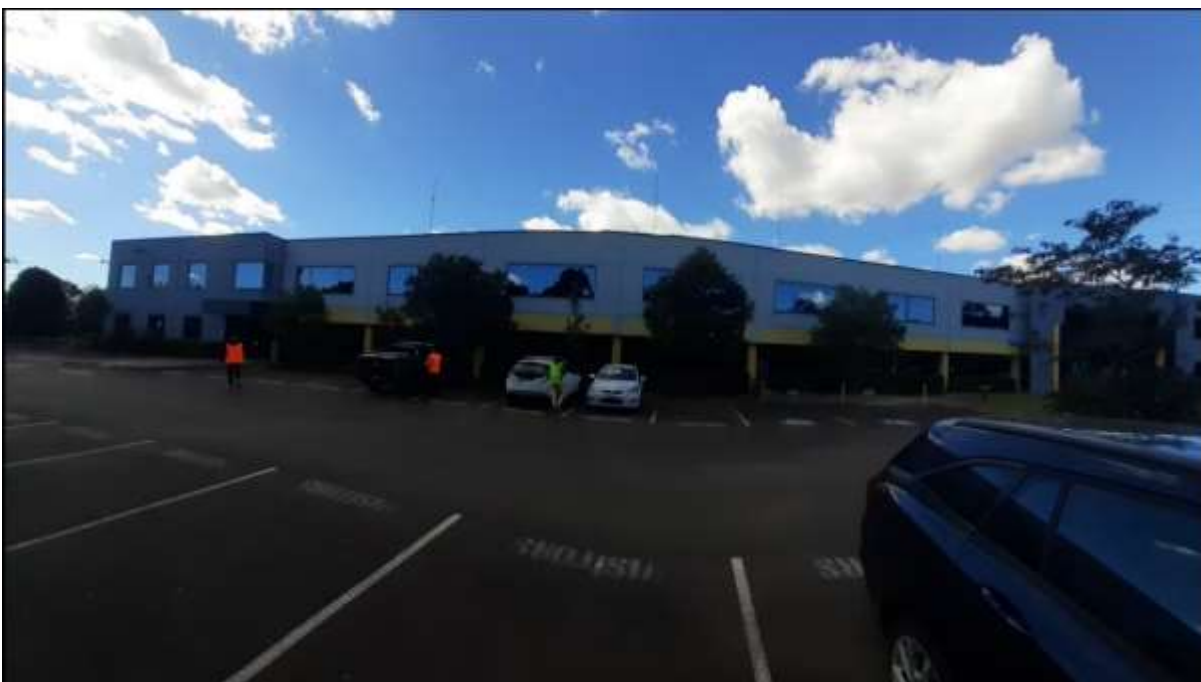
Figure 32: Existing office building west elevation
