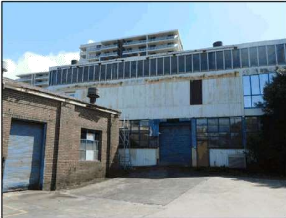
Figure 7: Southern side of southern building.
