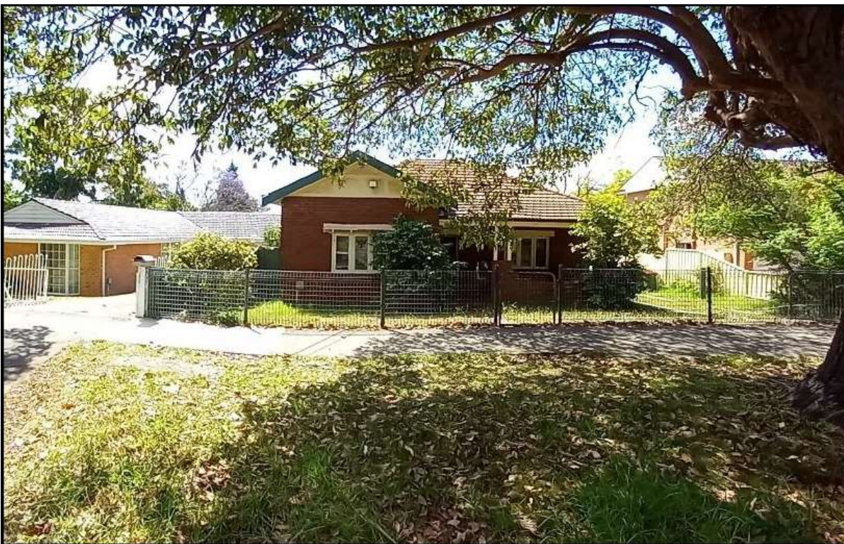
Figure 14: Existing dwelling at 3 Badgery Avenue
