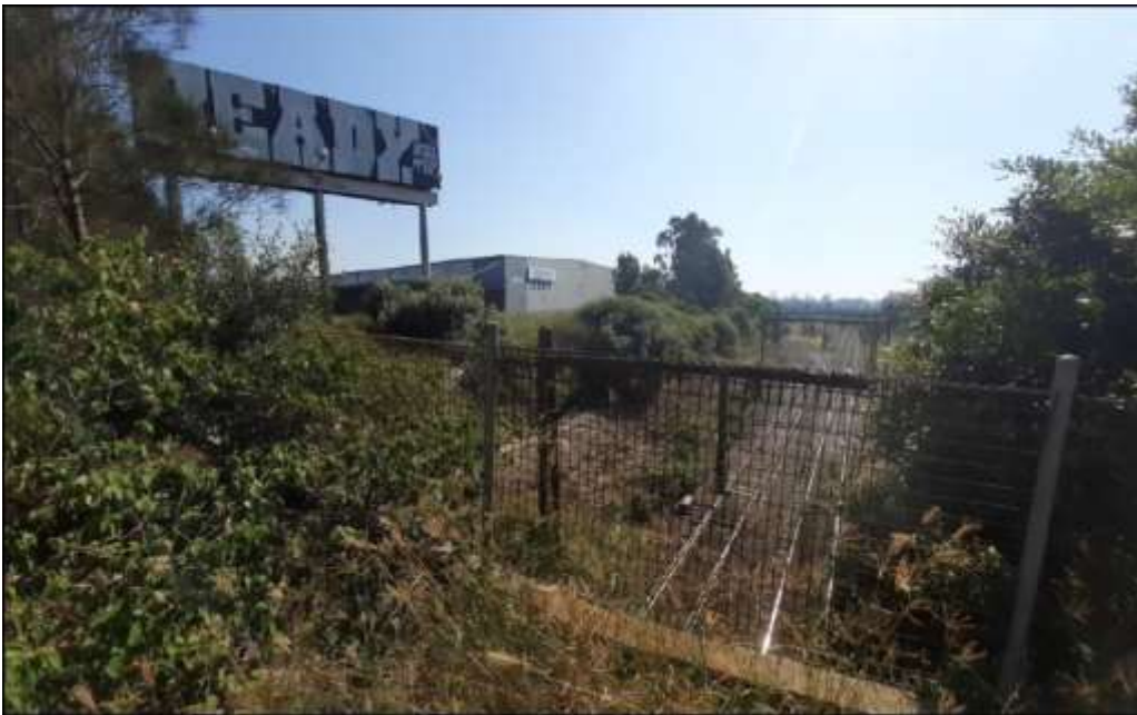
Figure 20: Subject site south-east elevation and adjacent railway tracks
