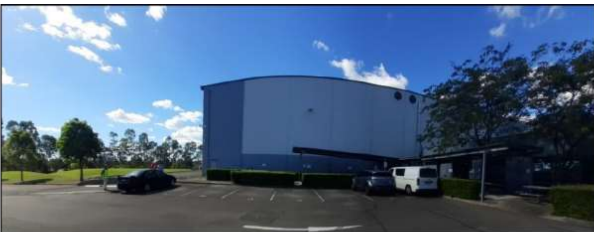
Figure 23: Existing warehouse west elevation (north end) to be retained
