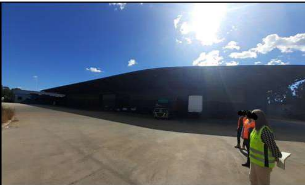
Figure 27: Existing warehouse loading bay (south elevation)
