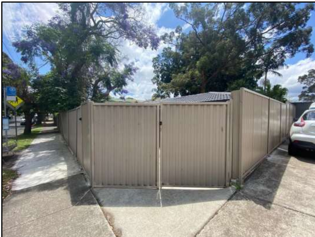
Figure 28: Existing internal and secondary frontage solid fencing – separating secondary dwelling and dwelling house.
