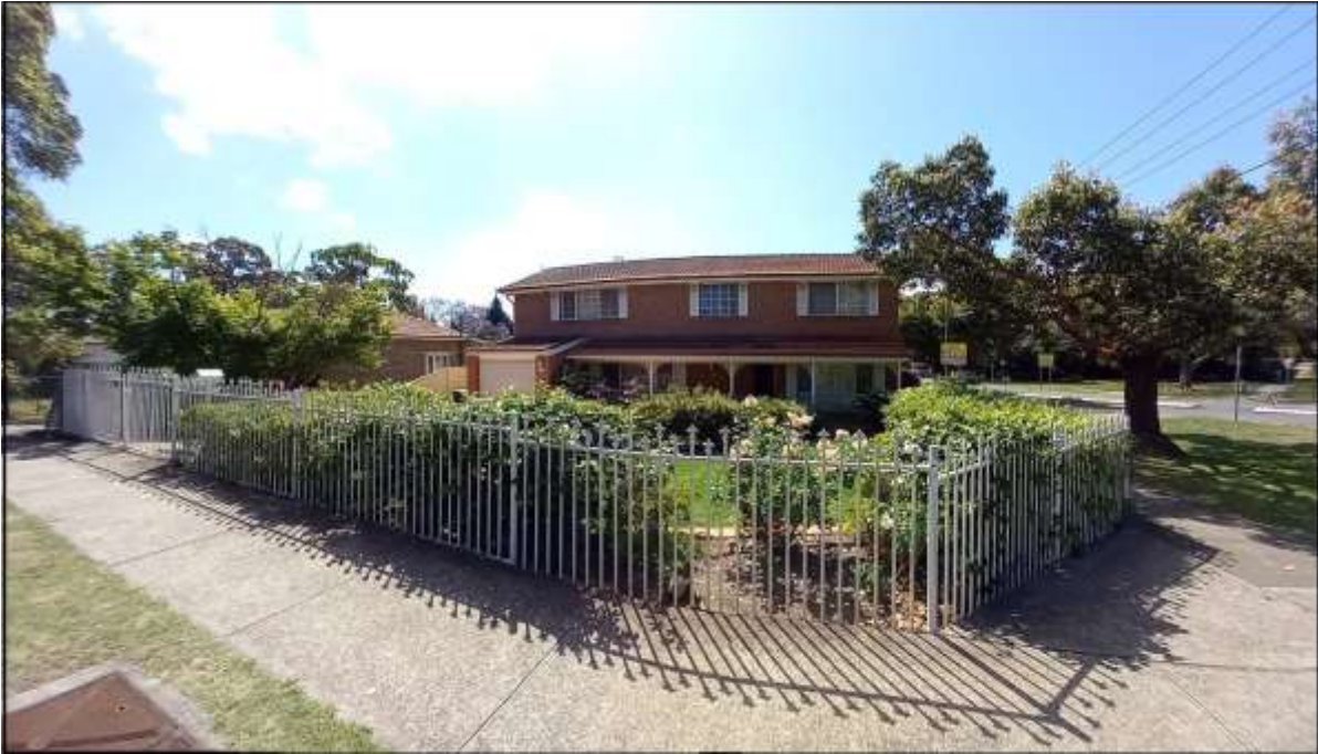
Figure 13: Existing dwelling at 1A Badgery Avenue
