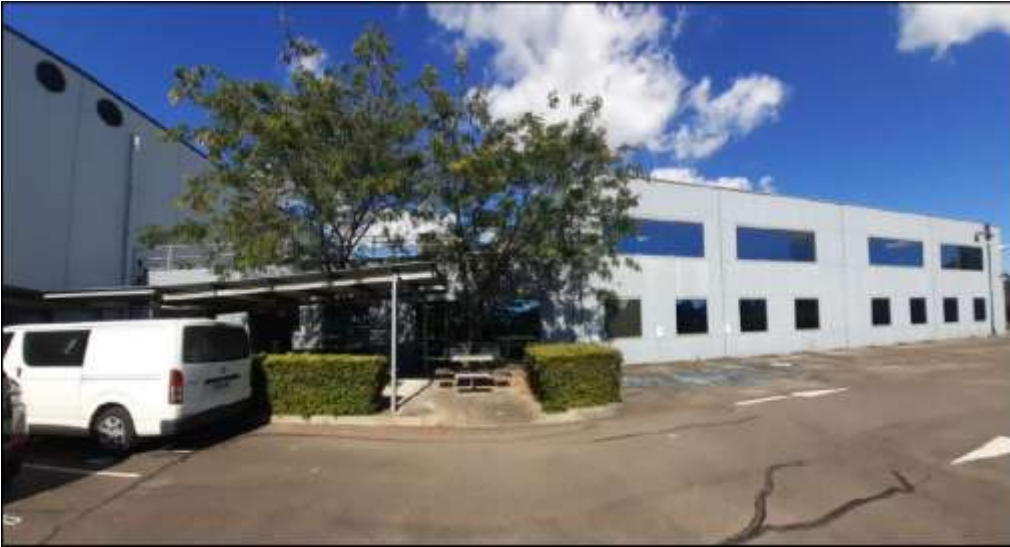
Figure 21: Existing two-storey office (right) to be demolished
