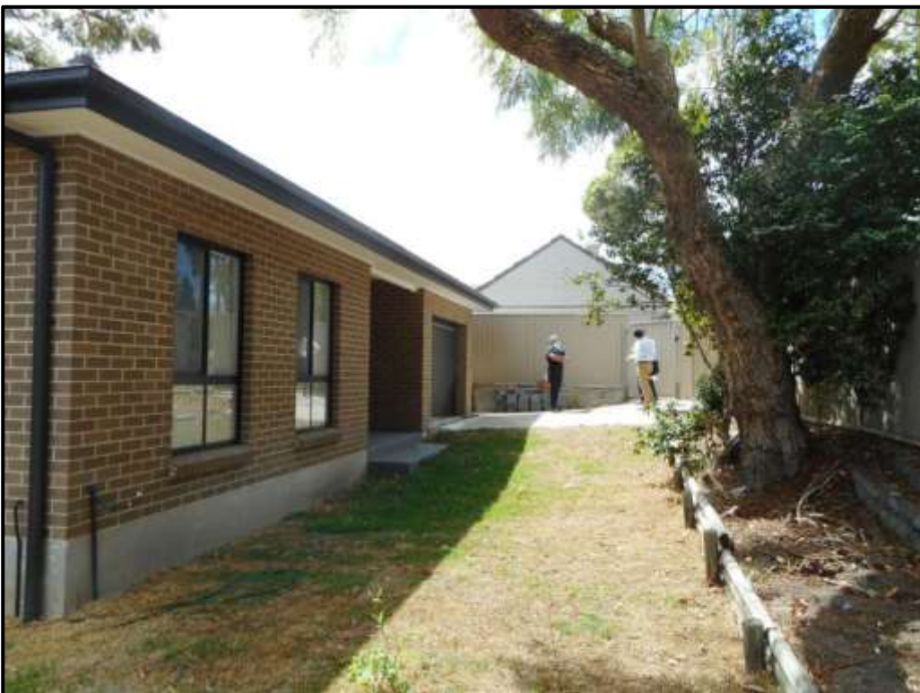
Figure 21: Open area to the south of the secondary dwelling and showing area for access ramp into front door
