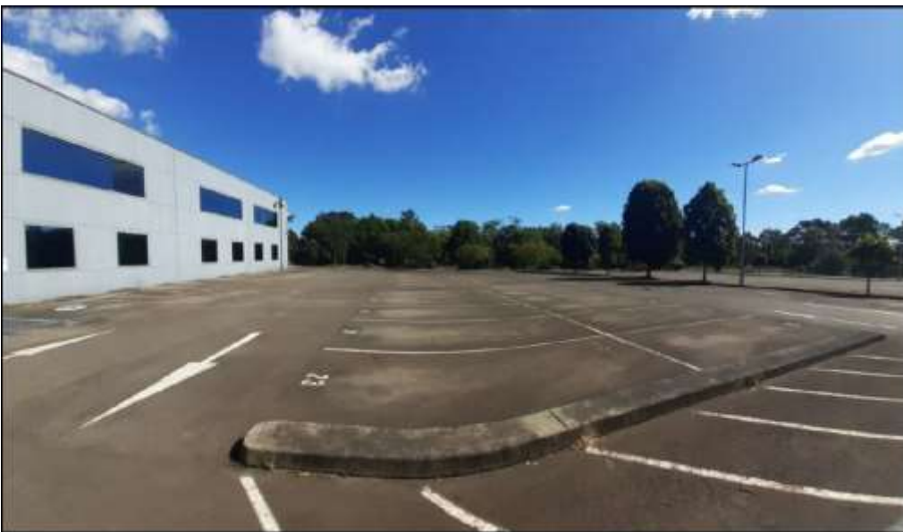
Figure 22: Existing office and northern carpark to be demolished (west-facing)
