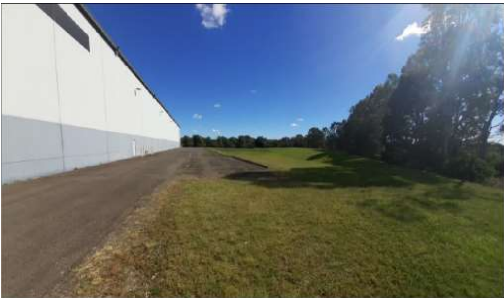
Figure 36: Existing warehouse and northern bounds (west-facing)
