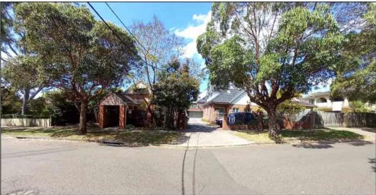
Figure 18: Adjoining streetscape 31 Mackenzie Street & 40 Bates Street (Bates Street side)
