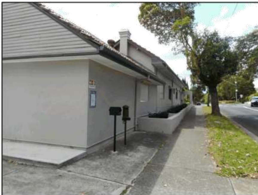
Figure 27: Secondary frontage of dwelling house – addressing Albyn Road
