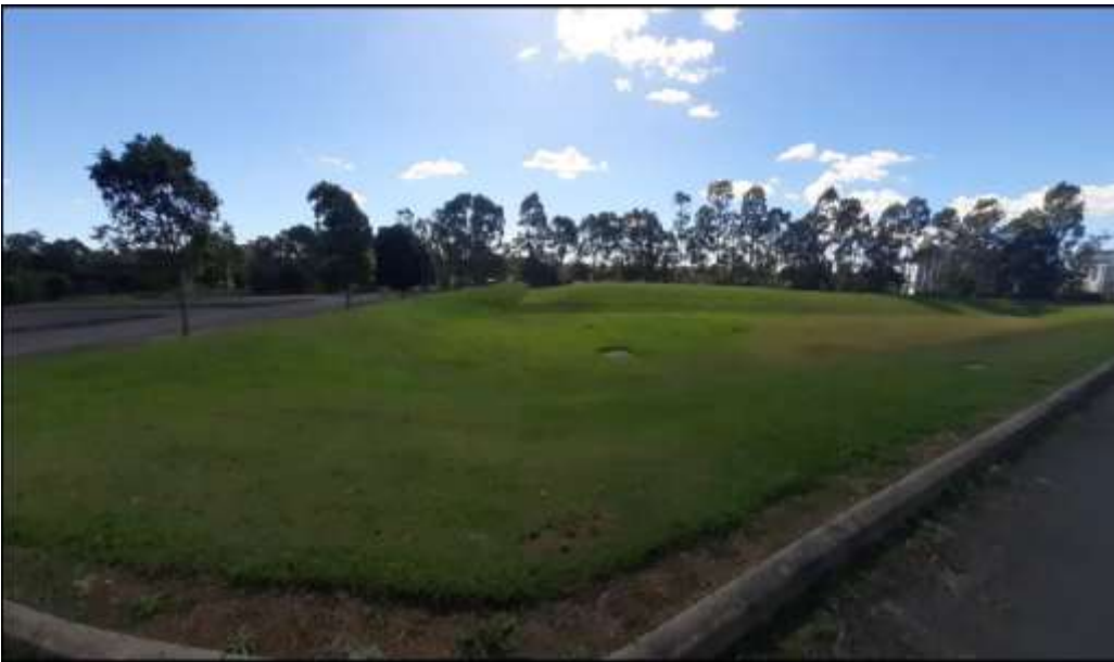
Figure 25: Existing on-site detention basin and north boundary
