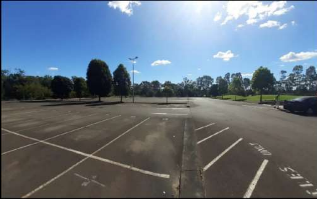
Figure 24: Existing north carpark to be demolished (north-facing)
