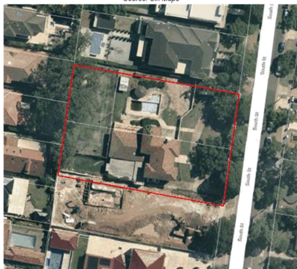
Figure 2: Aerial View of 19-21 South Street Source: Maps
