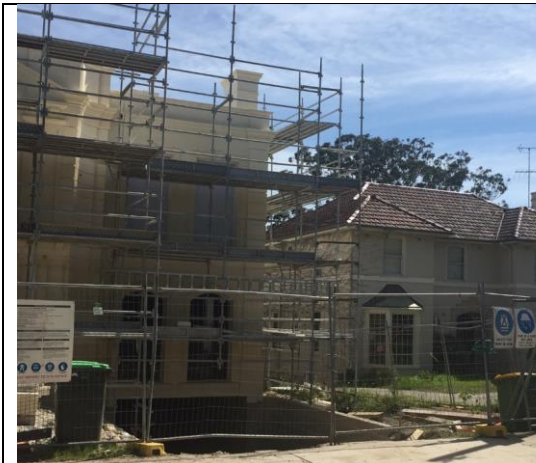
Figure 9: 23 South Street, currently being constructed.
