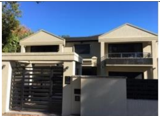
Figure 7: North: Two (2) storey rendered brick dwelling house at 17 South Street.
