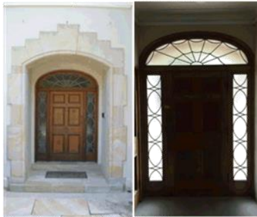
Figure 15: Front Door Source: POC+P Architects
