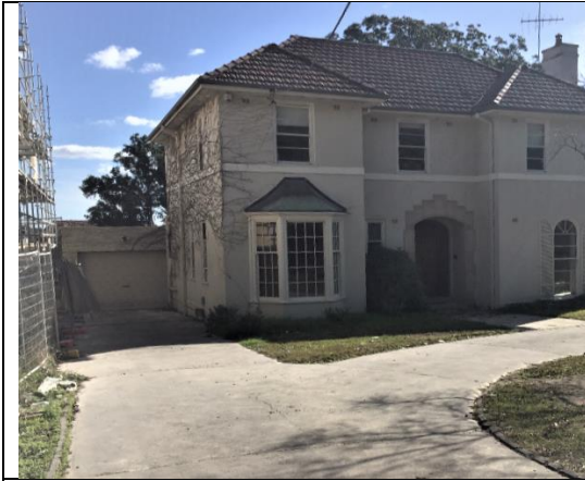
Figure 3: (2) storey 'Georgian Revival' rendered brick residence on the southern-most lot (Lot 66)
