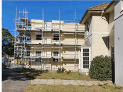
Figure 25: 23 South Street, Under Construction Source: POC+P Architects 2020
