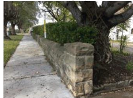
Figure 6: Fence at Vehicular Entrance Facing South Source: Urbis
