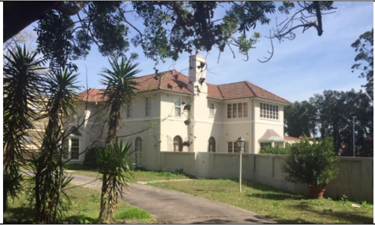
Figure 4: View to the Northern Elevation and garden fence of the 'Georgian Revival' rendered brick residence.
