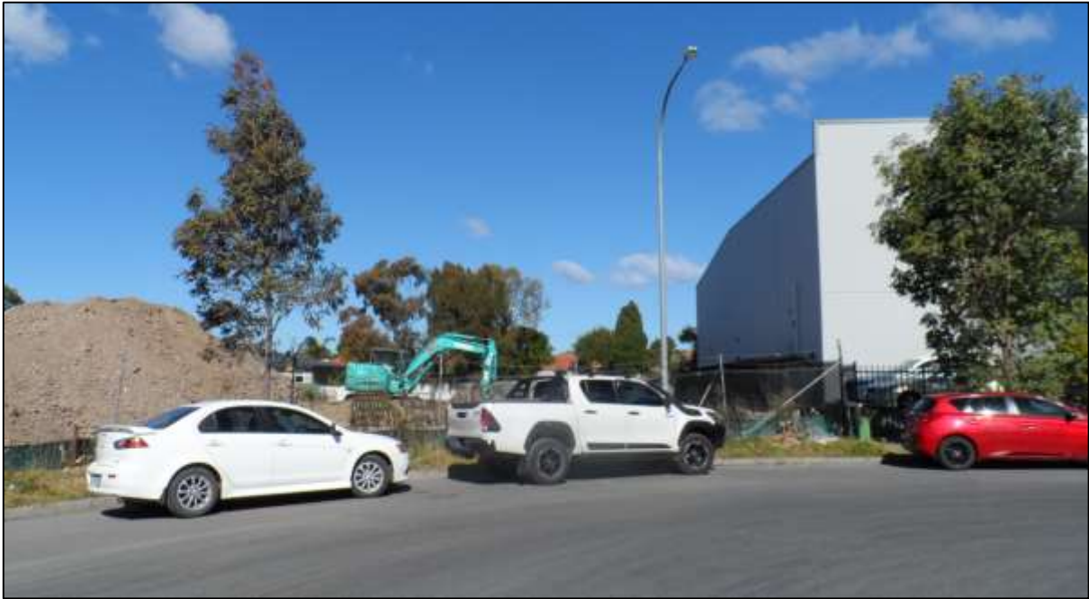
Figure 4: Southerly view from Bellfrog Street of the subject site.
