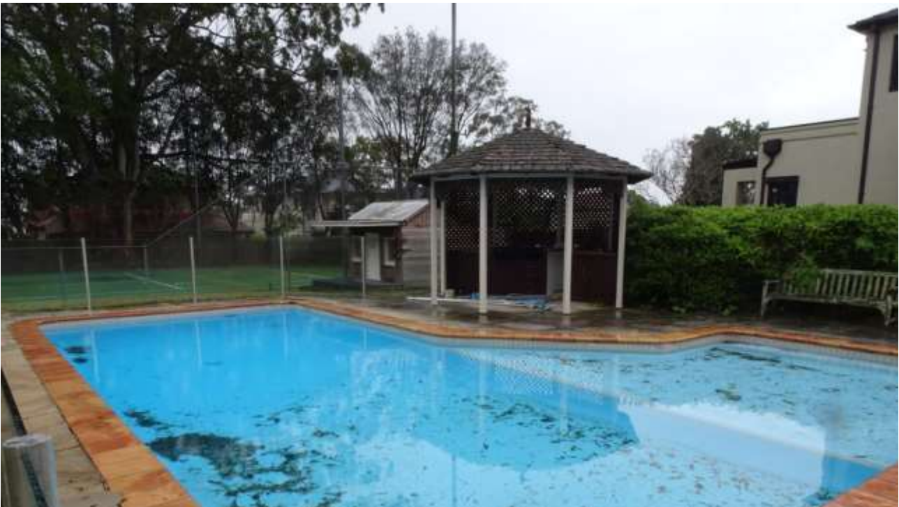
Figure 10. Swimming pool and detached timber cabana structure (c. 1987-1988).
