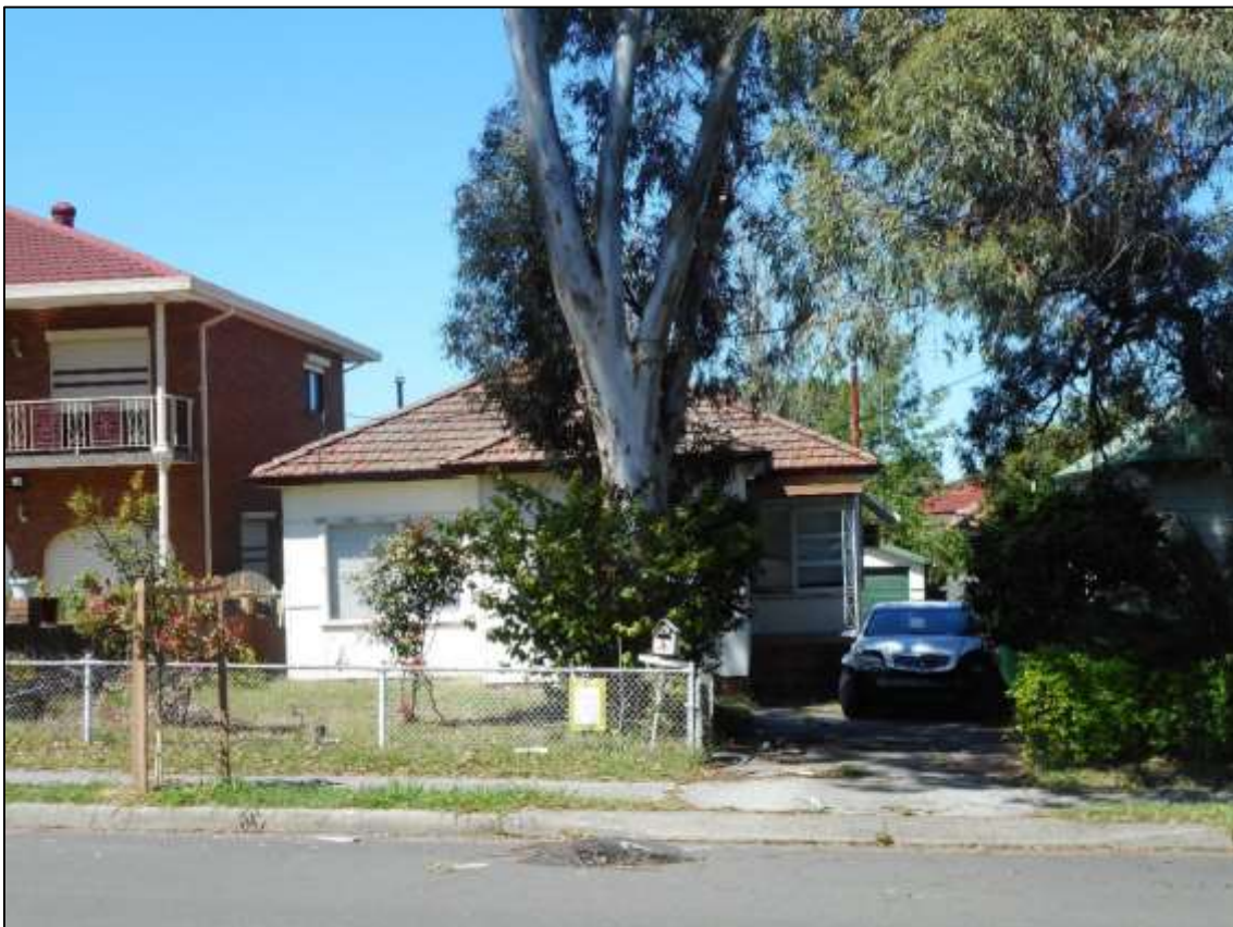
Figure 2: No. 12 Therry Street East, Strathfield South
