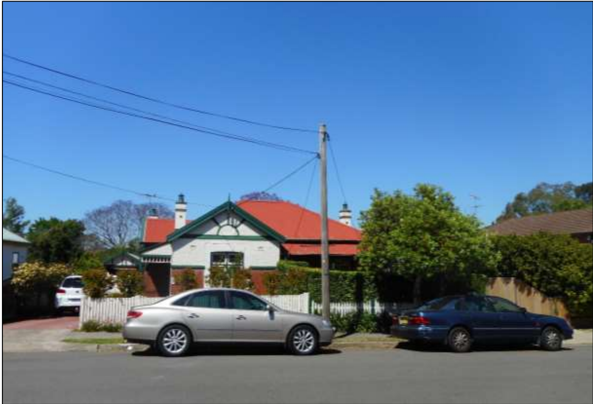
Figure 7: Semi-detached dwellings at No. 16 and 18 Therry Street East, Strathfield South
