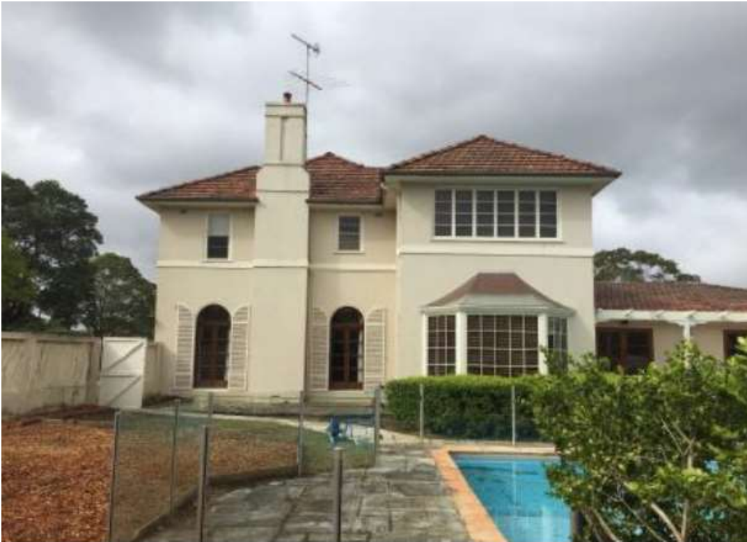
Figure 7. Northern side elevation of the existing building (Source: Urbis).
