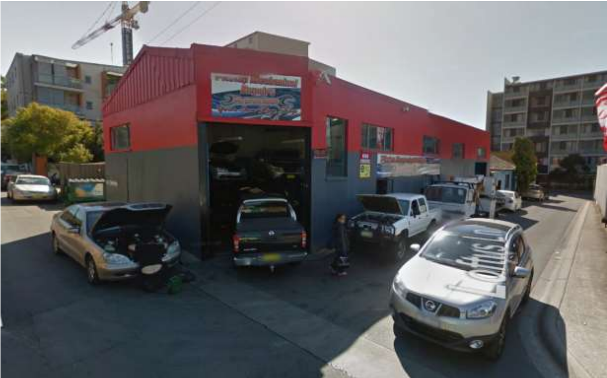
Figure 3: Westerly view of the subject site from Loftus Lane
