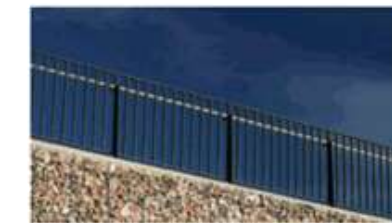
METAL BALUSTRADE TO VOIDS / CORRIDORS
