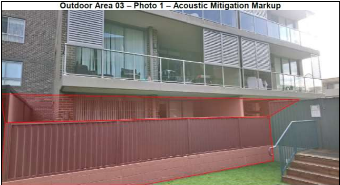
Figure 8: Proposed acoustic barrier and roof structure as recommended in the revised acoustic report facing north.
