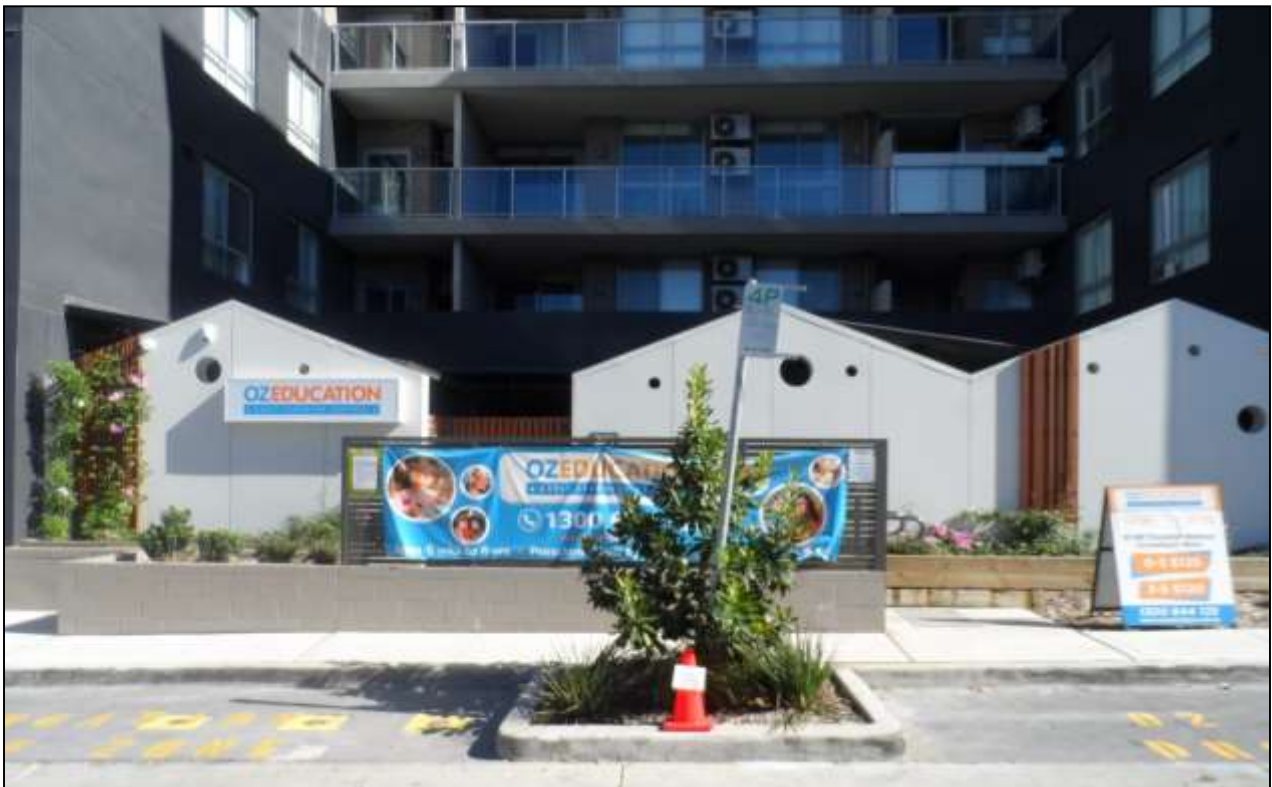
Figure 2: View of the existing child care centre from Courallie Avenue.
