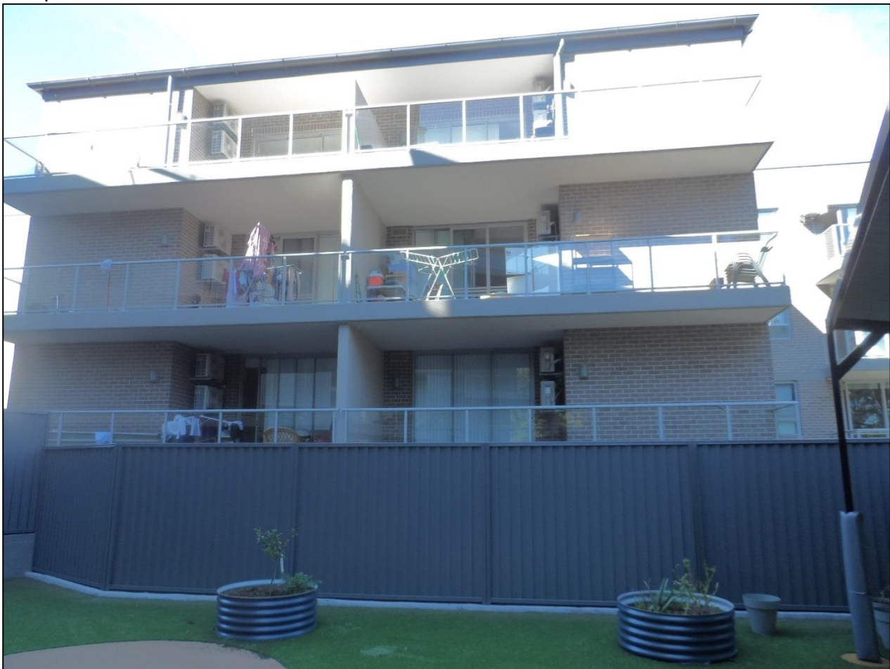
Figure 4: Outdoor play area 03 and nearby residential units.
