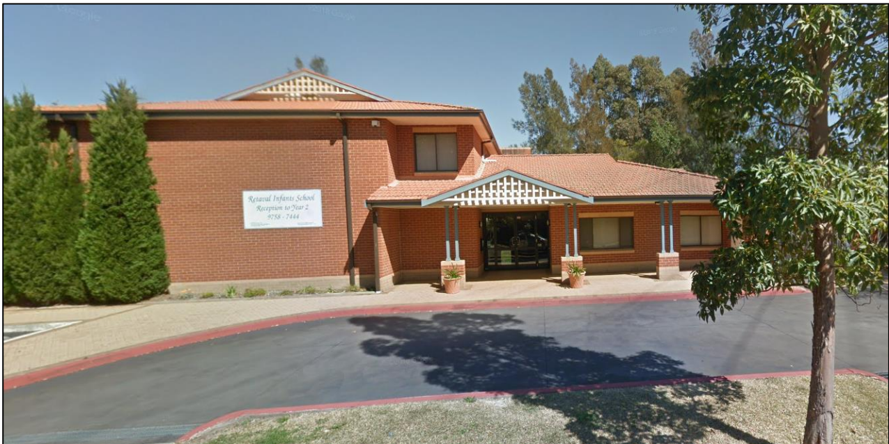
Figure 2: View of the existing infant school from Elliott Street.
