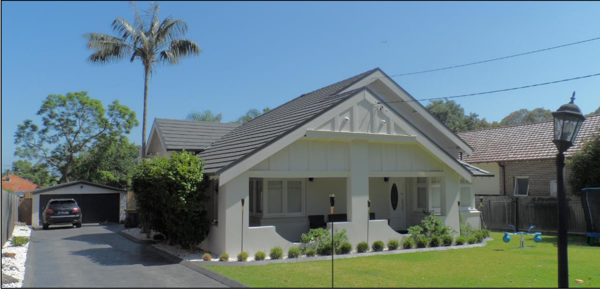
Figure 3: Front façade of the subject site at 47 Merley Road, Strathfield.
