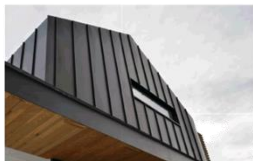
MC FLAT PAN STANDING SEAM METAL CLADDING COLORBOND 'MONUMENT'
