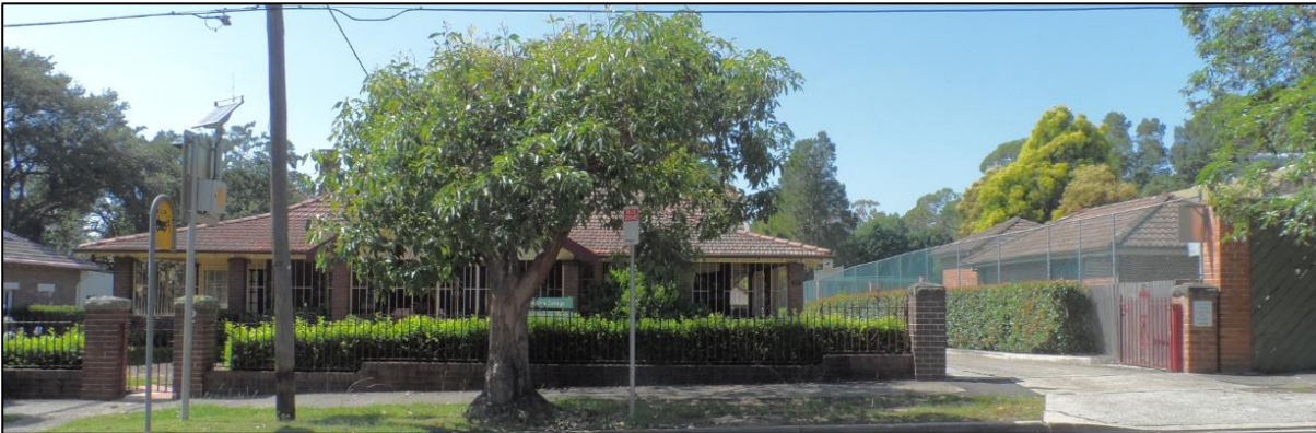
Figure 4: View of 22 Merley Road apart of St Patrick's College directly opposite the site.
