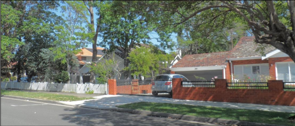
Figure 6: View of adjoining neighbours at 49 and 51 Merley Road, Strathfield.
