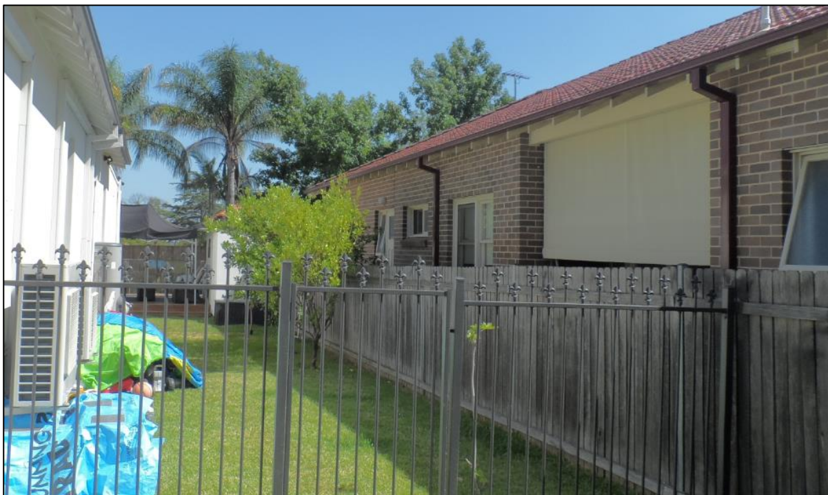
Figure 11: View of existing windows and courtyard of 45 Merley Road facing west.
