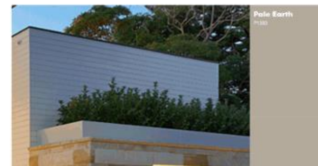
FC EXPRESSED HORIZONTAL JOINT FC CLADDING DULUX 'PALE EARTH'
