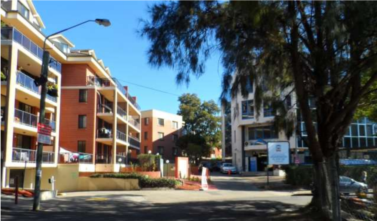
Figure 4: View of the site and adjoining residential flat building from The Crescent.
