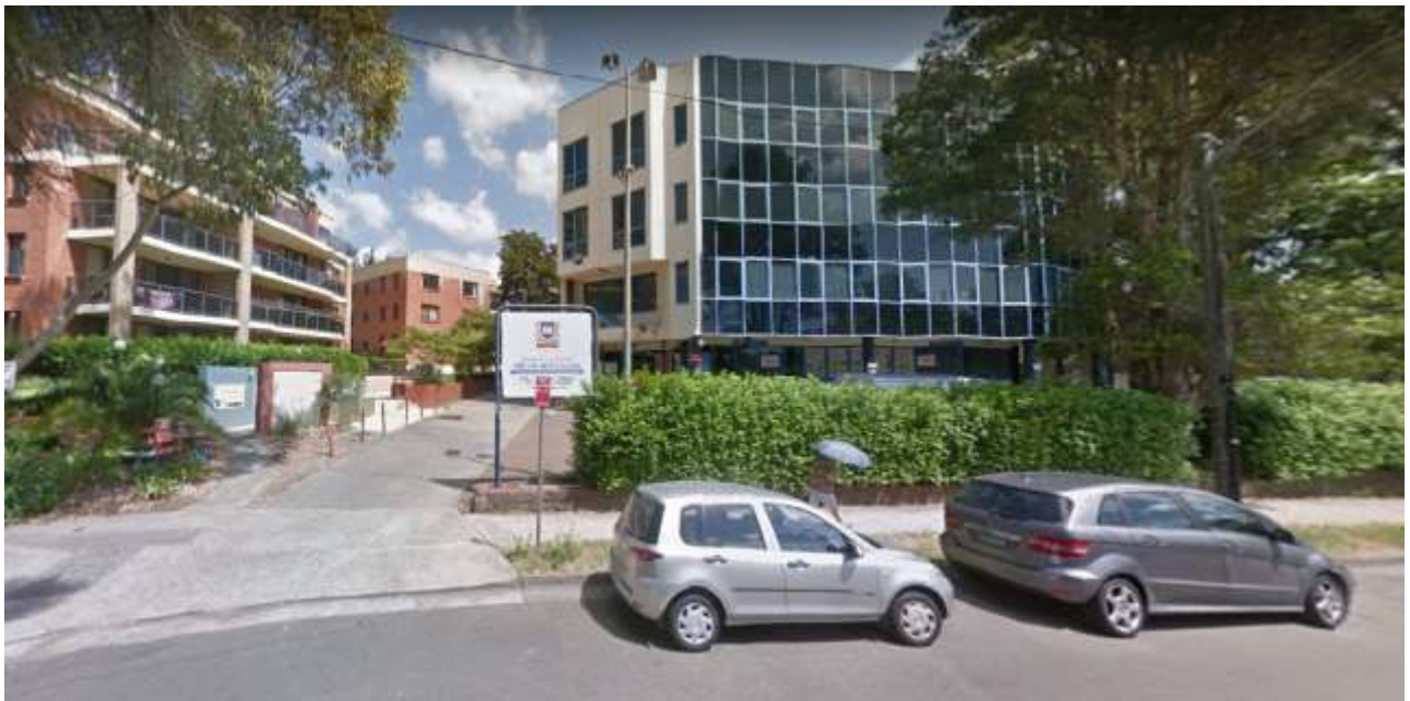
Figure 2: The site as viewed from The Crescent.
