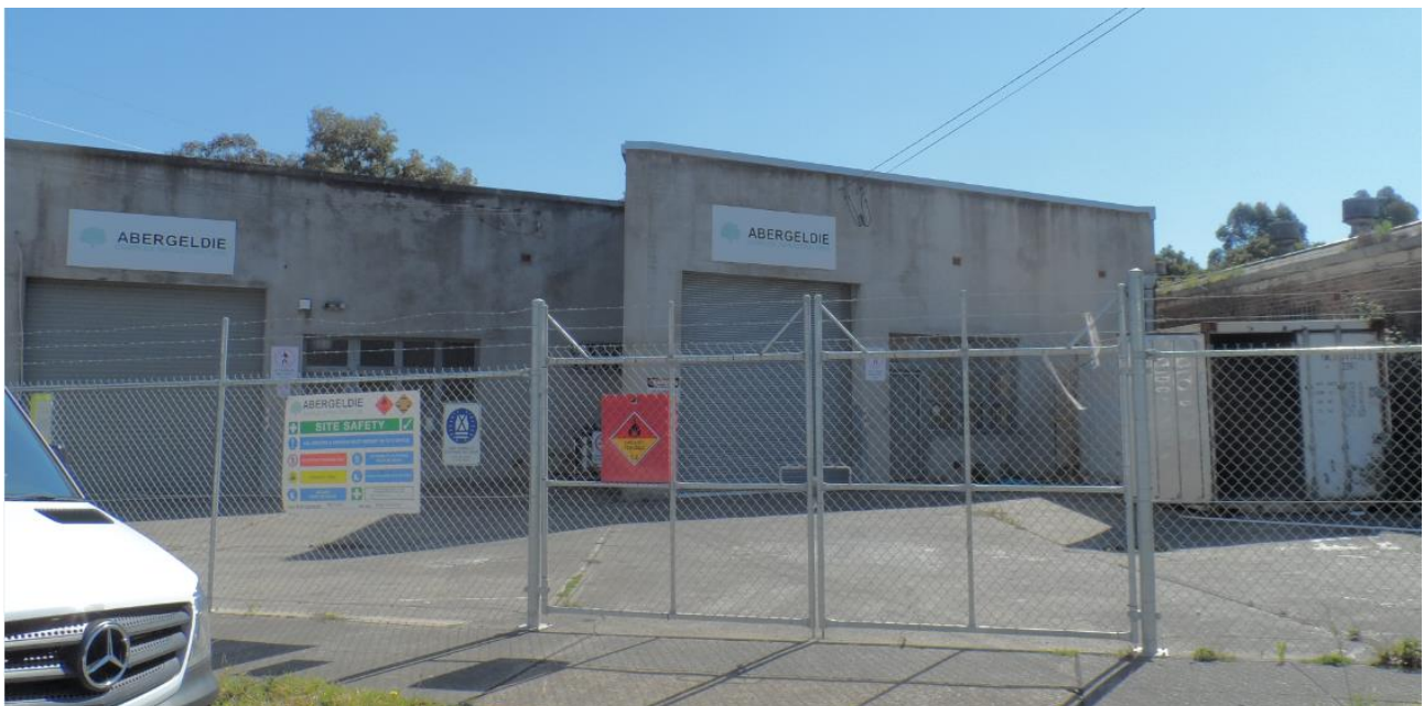
Figure 2: View of the subject site from Dunlop Street.
