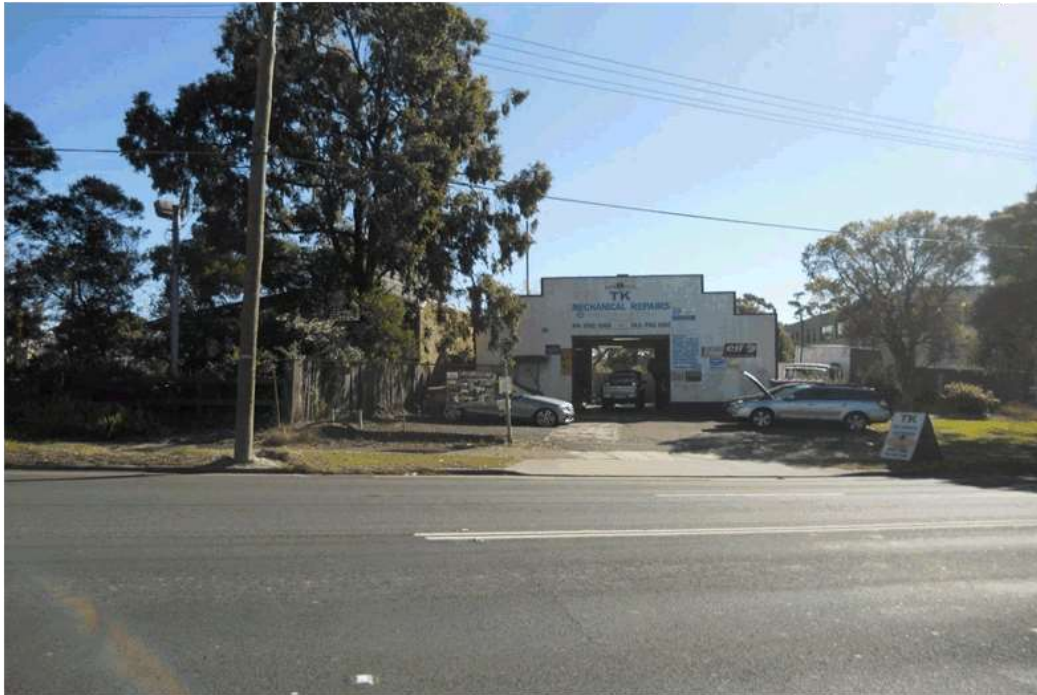
Figure 12 View North Towards Adjoining Site – Mechanical Repair Premises - 27 -35 Punchbowl Rd
