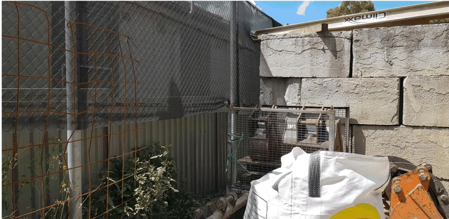
Figure 20 - Stone Block Wall off Boundary
