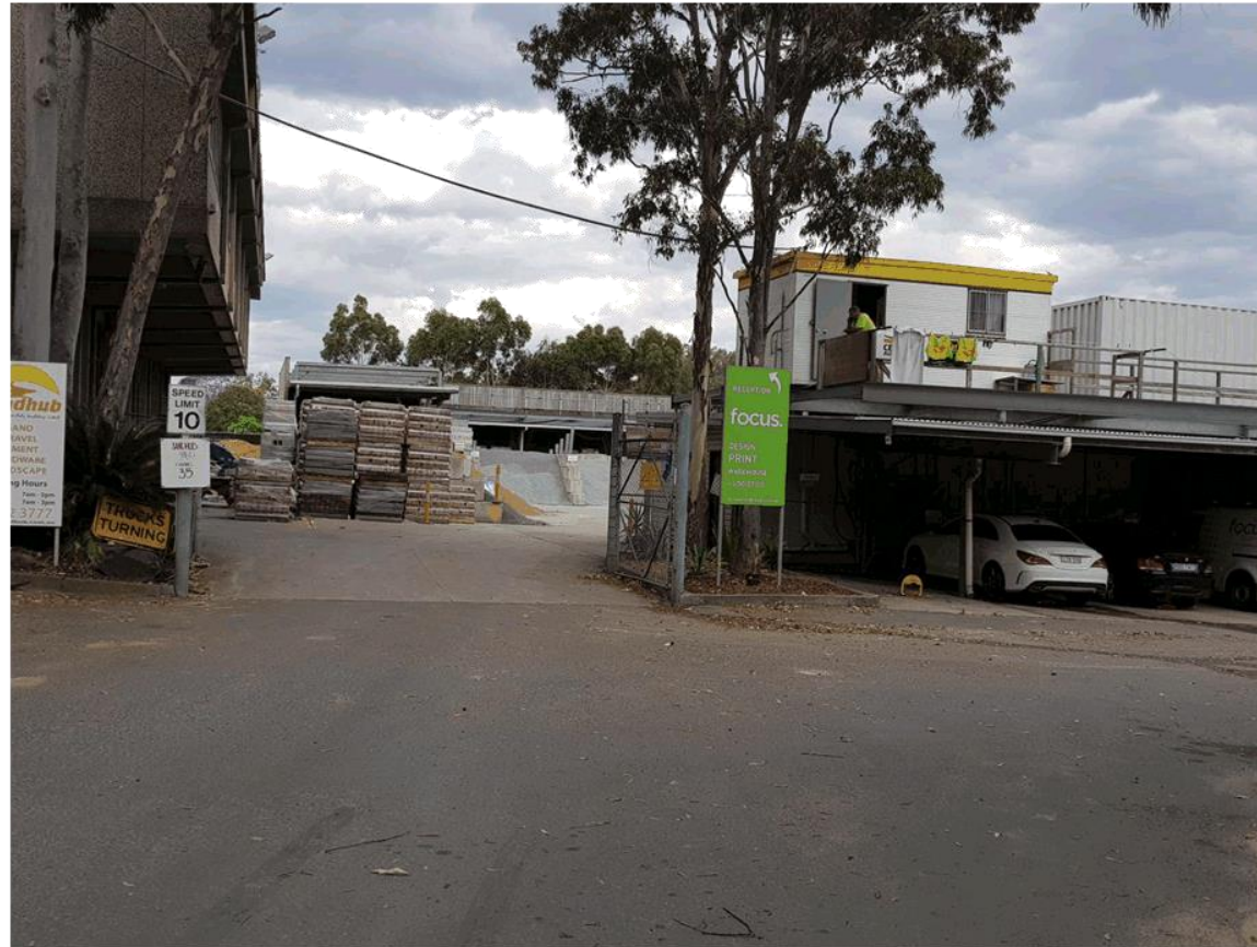
Figure 10 – Entry to Site
