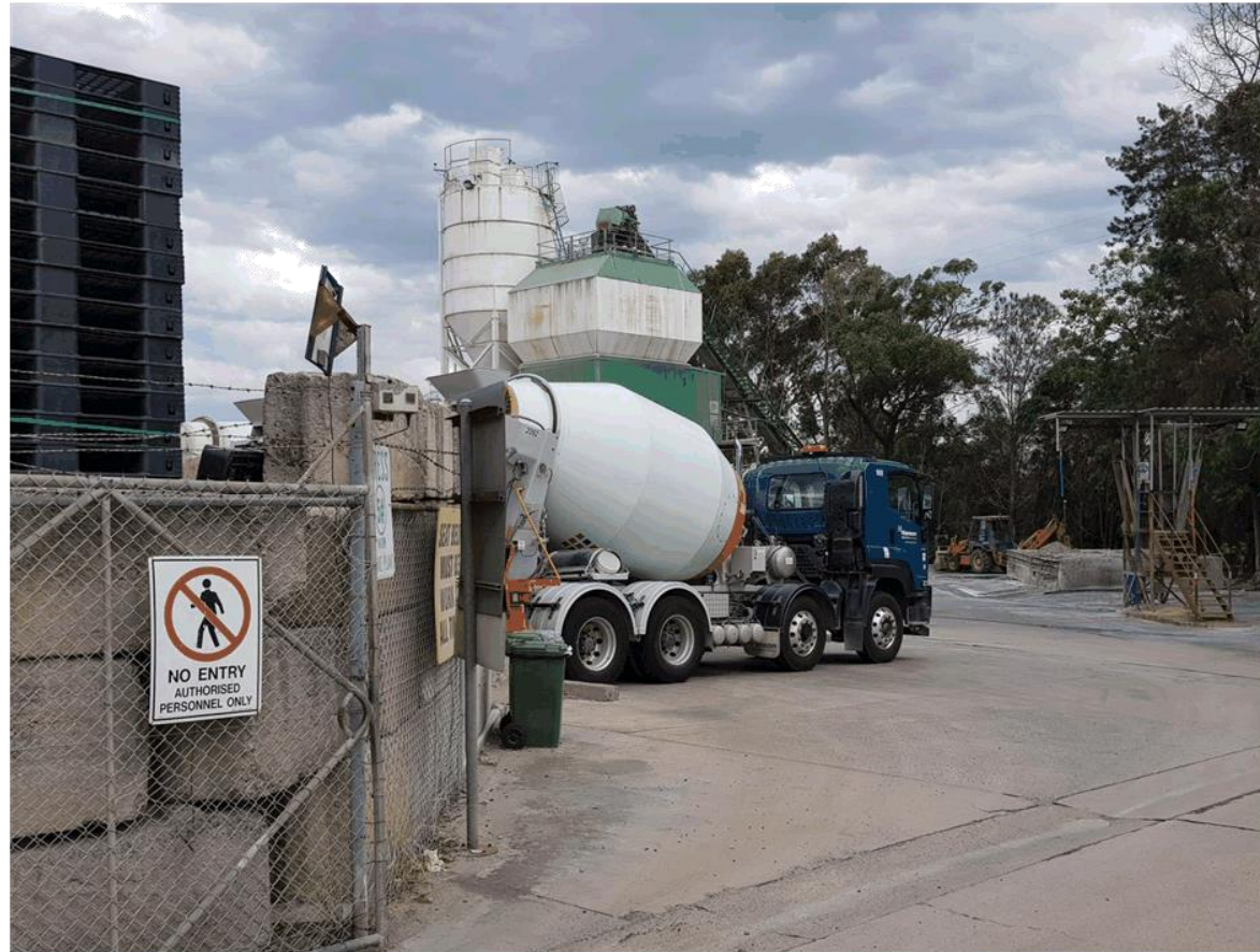
Figure 4 - Hanson Concrete Batching Plant
