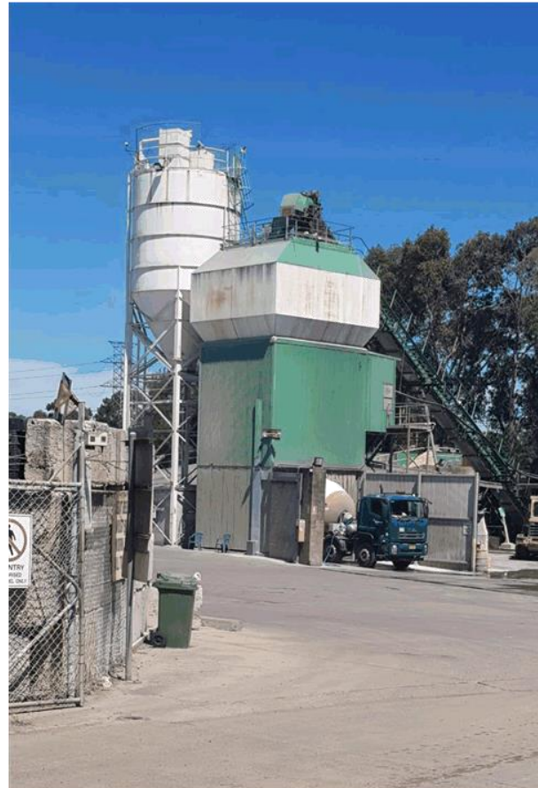
Figure 5 – Hanson Concrete Batching Plant
