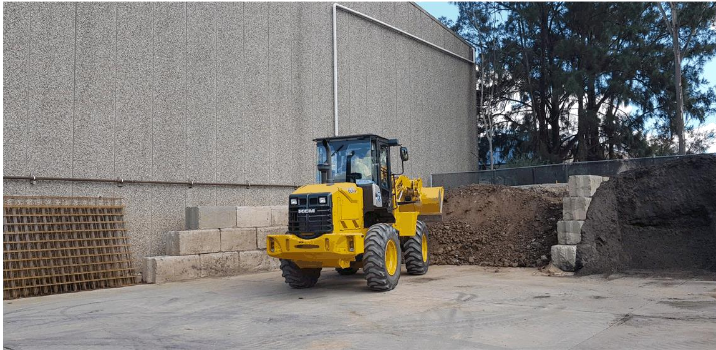
Figure 19 - Access to Storage Material in Northern Corner
