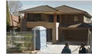
(13) 37 MYRNA ROAD DOUBLE STOREY BRICK RESIDENCE + TILED ROOF - ADJOINING DWELLING TO THE NORTH OF SUBJECT SITE
