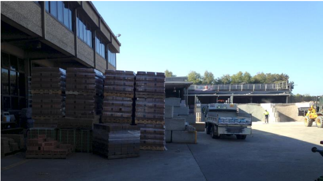
Figure 3: View inside subject premises.
