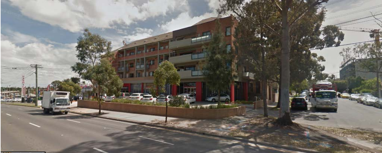
Figure 2: View of the existing commercial tenancy from Parramatta Road.
