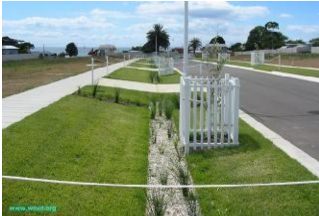
Figure 3. Example of Grassed swale (Source: Water Sensitive Urban Design of the Sydney Region)
