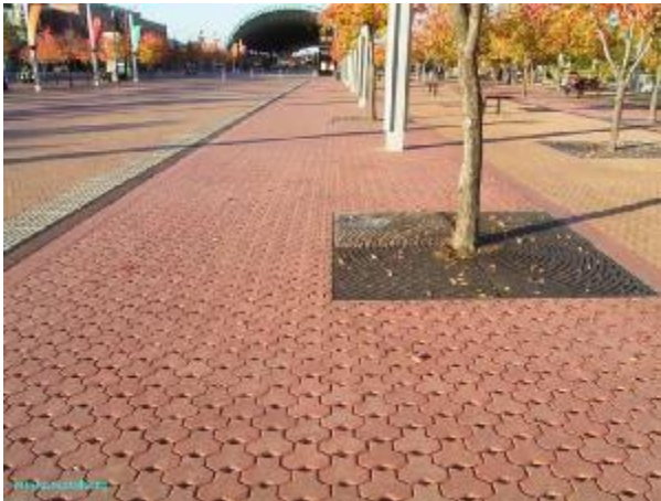
Figure 6. Example of Porous Pavement (Source: Water Sensitive Urban Design of the Sydney Region)
