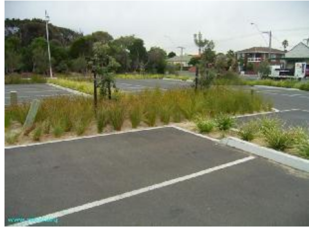
Figure 7. Example of Porous Pavement surrounding carparks (Source: Water Sensitive Urban Design of the Sydney Region)
