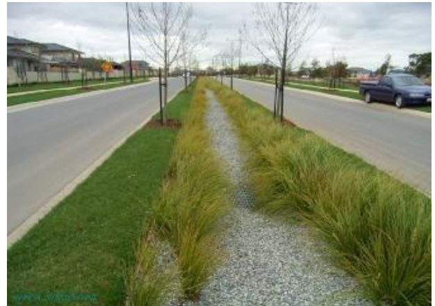
Figure 4. Example of Vegetated swale (Source: Water Sensitive Urban Design of the Sydney Region)
