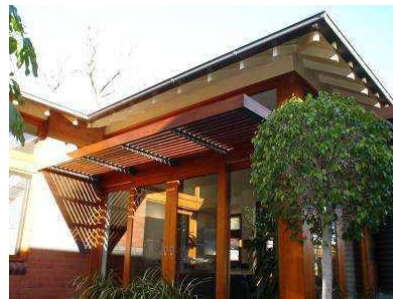
Figure A.18 - Provide louvred sunshade devices to provide filtered sunlight particularly in winter.
