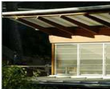
Figure A.19 - Window shades can be used as a natural cooling strategy.
