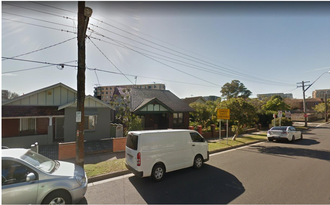
Photograph 1: Shows the site as viewed from Loftus Crescent.
