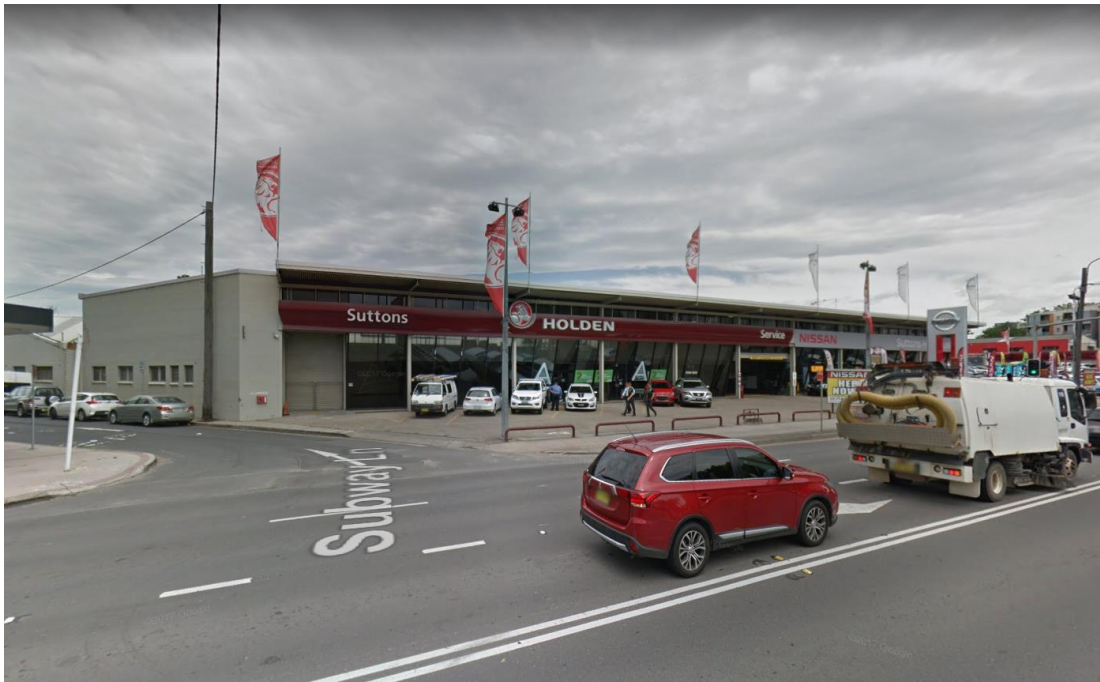
Photograph 6: Shows a Holden dealership, which neighbours the site on its northern boundary.
