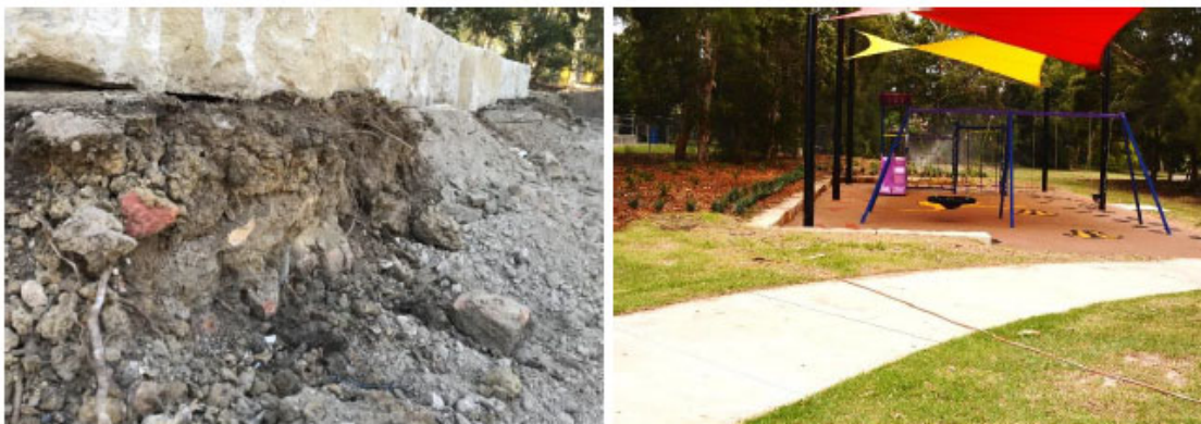
Monitoring of works and New Playground with Aboriginal flag theme
