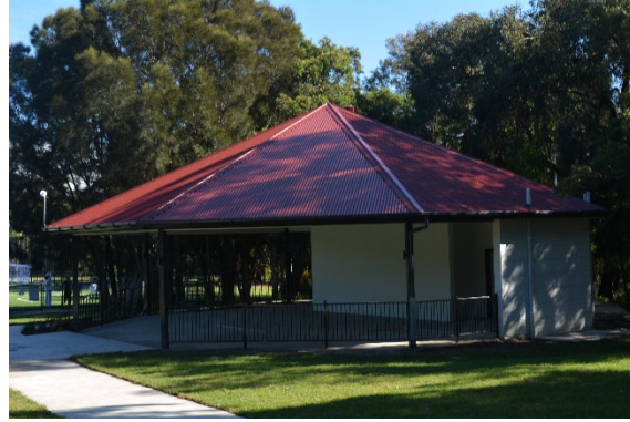
Amenities building (near Homebush Rd) built in 2022 and rated Excellent
