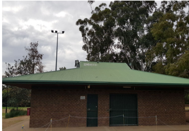
Amenities building (former) is rated as Good.
