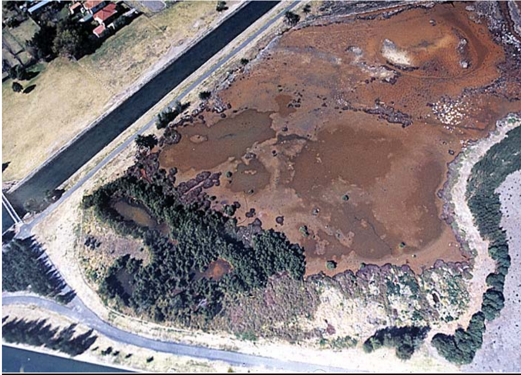
Mason Park from the air, 1995. Large areas are mudflat. Acid levels in the soils have limited growth. The current tidal inlet is adjacent to the mangroves in the bottom left corner of the photo. The proposed new inlet is to be situated at top left of the saltmarsh at a point where the distance to the concrete estuary channel widens.
