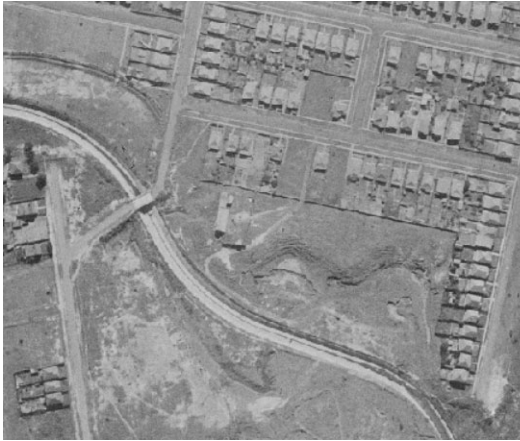
Southend Tennis Centre aerial photograph (1947)
