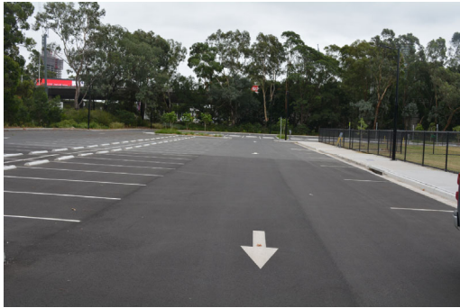
Bressington carpark was built in 2018 and is assessed as excellent condition.
