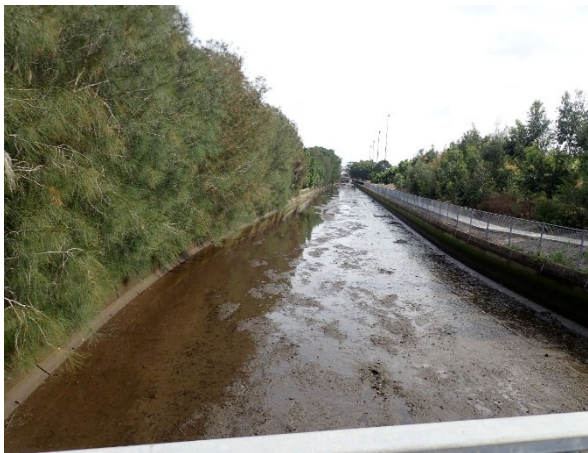
Figure 31 Saleyards Creek is now a concrete lined channel with a cycle track and revegetation planting in Bressington
