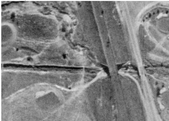
1943 Cooks River Freshwater Park and S Strathfield Golf Course (east) bisected by the railway. Source: SIX Maps
