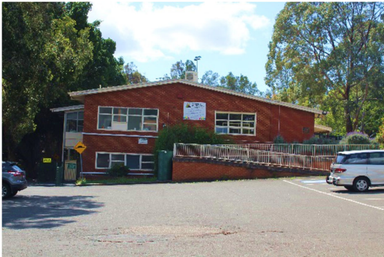
Strathfield Children's Centre – Fraser Street
