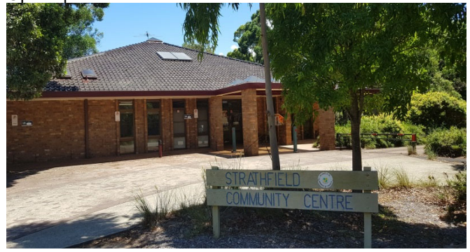
Strathfield Community Centre – Bates Street
