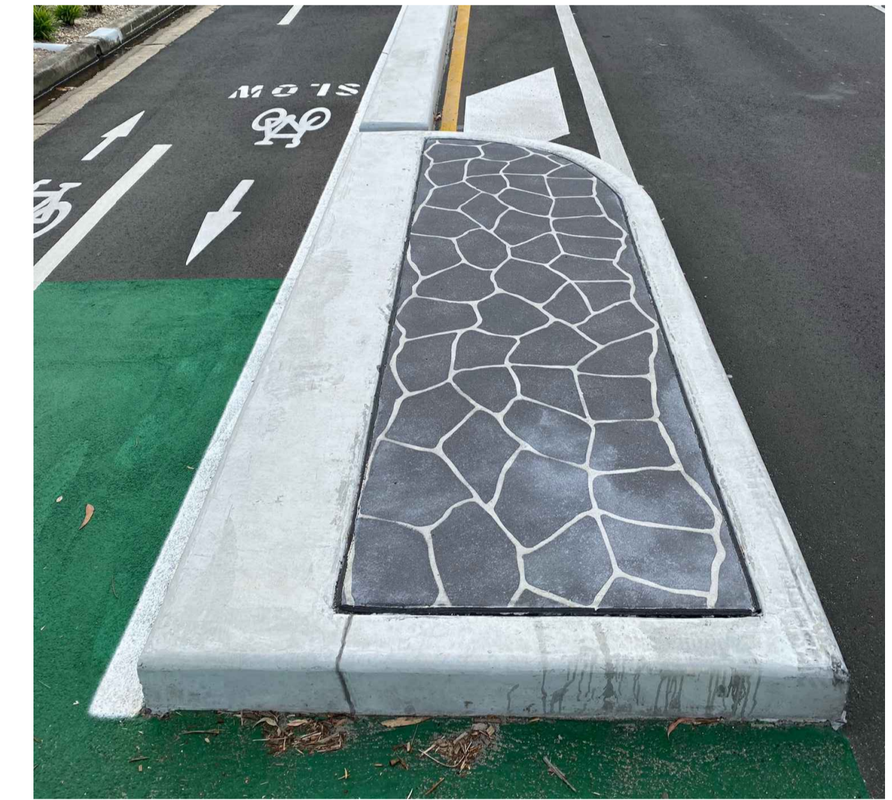
Example of stencil pattern (different colour shown)
