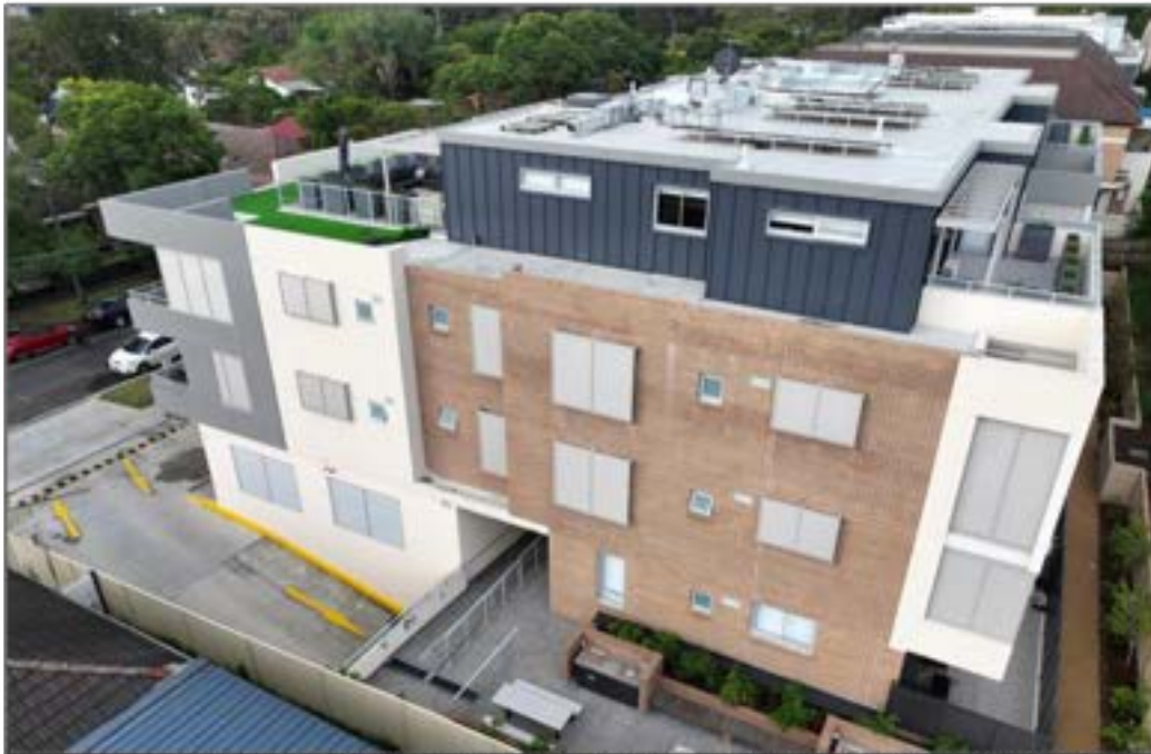
Figure 28: Drone photograph showing privacy screens on 28 Courallie Avenue facing the subject site
