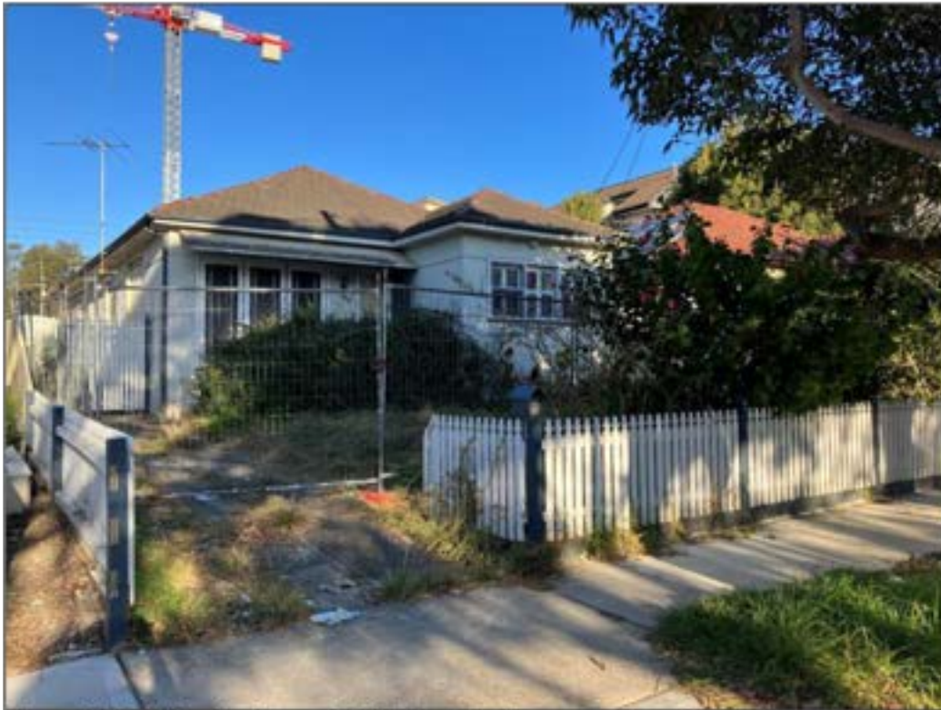
Figure 15: Existing development at 30 Courallie Avenue, as viewed from the street
