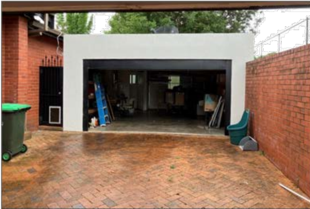
Figure 26: The garage on the subject site
