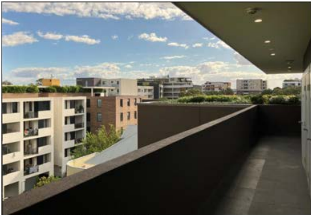
Figure 11: Open breezeway within Building B
