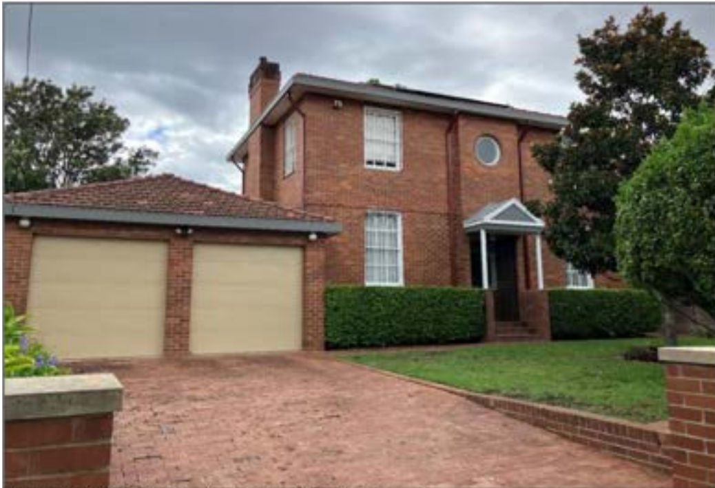
Figure 30: 14 South Street, as viewed from the street
