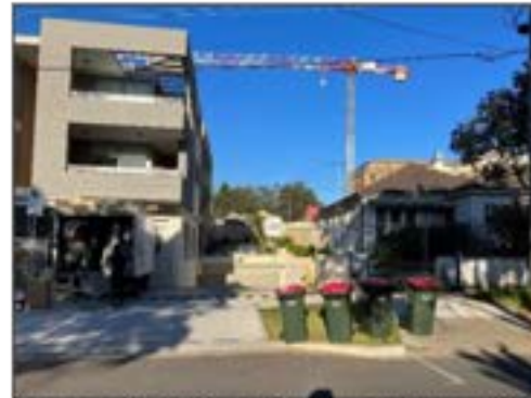
Figure 18: The interface between 28 Courallie Avenue and the subject site, showing the basement ramp
