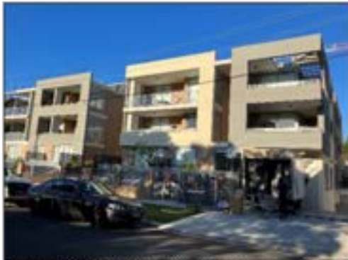
Figure 17: 28 Courallie Avenue, as viewed from the street
