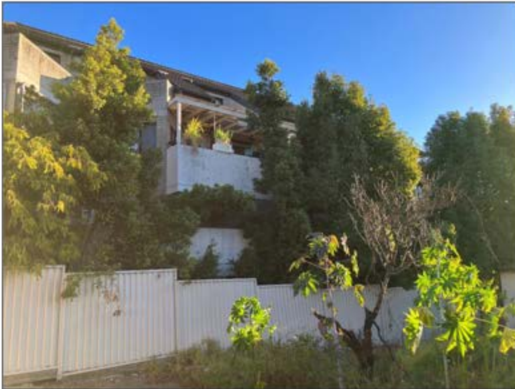
Figure 29: The northern side elevation of 34-36 Courallie Avenue, as viewed from the rear yard of the subject site
