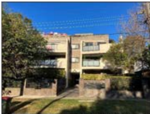
Figure 19: 34-36 Courallie Avenue, as viewed from the street
