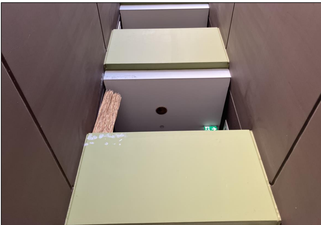
Figure 13: Temporary bamboo screening on one of the open breezeways
