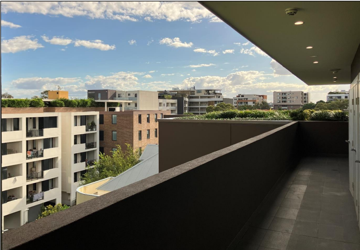
Figure 11: Open breezeway within Building B
