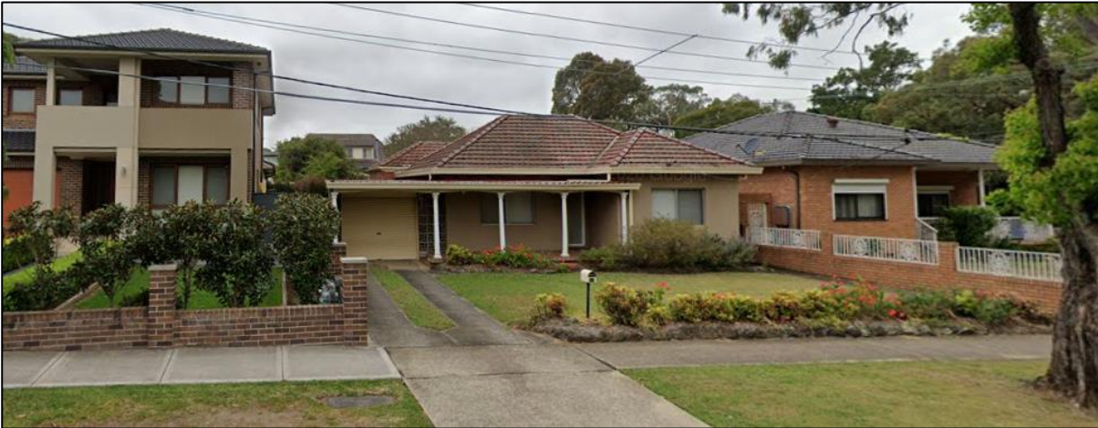
Figure 12: Subject site pictured centre. Adjoining dwelling at 30 Myee Avenue pictured left and southern adjoining dwelling at 28 Myee Ave pictured right.
