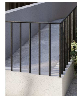
AL1 - DARK GREY VERTICAL METAL FENCING OR EQUIVALENT SIMILAR LOCATION: FRONT FENCE
