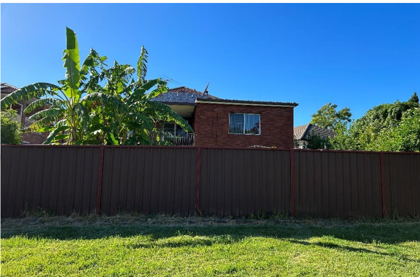
Figure 21: Looking east at No. 3 Highfield Crescent
