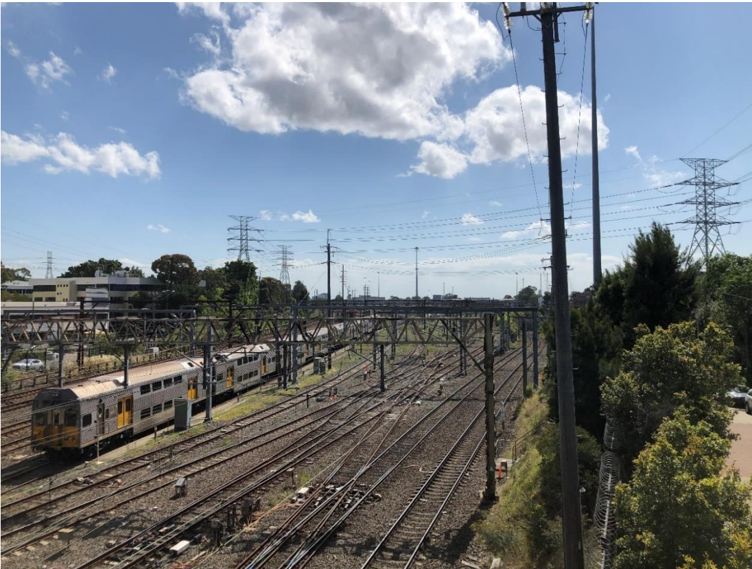
Figure 14 – The T1 and T2 rail lines located immediately south of the site
