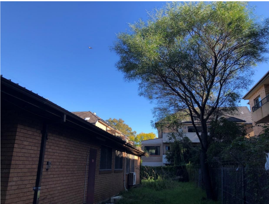
Figure 9 – On the left of the photo is the rear of the main structure at the site and on the right is adjoining development at 76-78 Courallie Avenue and 66-72 Marlborough Road
