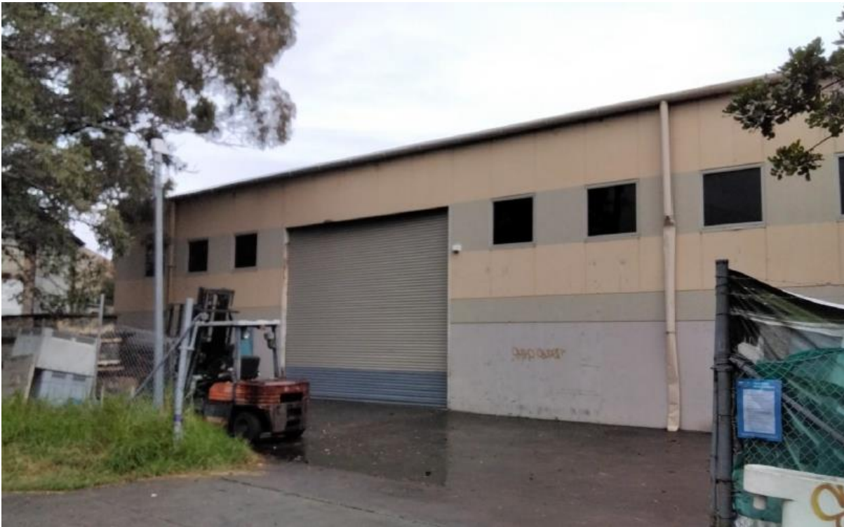
Figure 5. Front façade of the existing building on the site.
