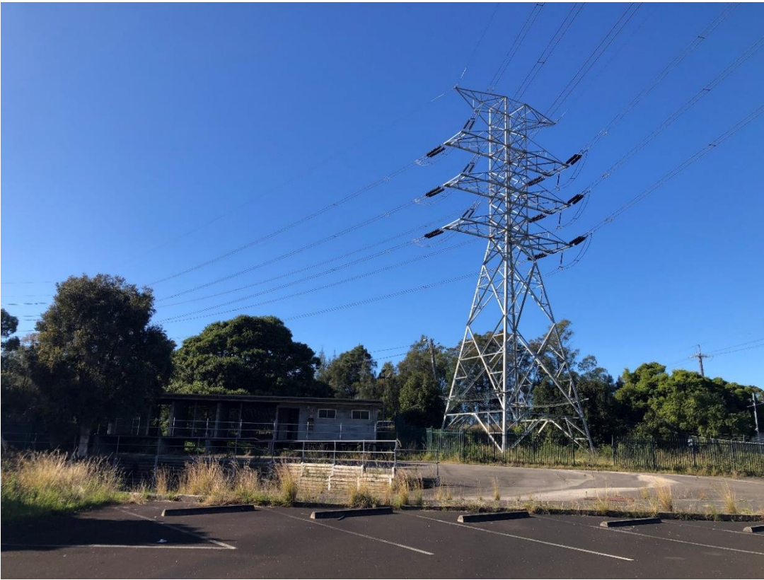
Figure 12 – The south eastern corner of the site where the transmission line is located
