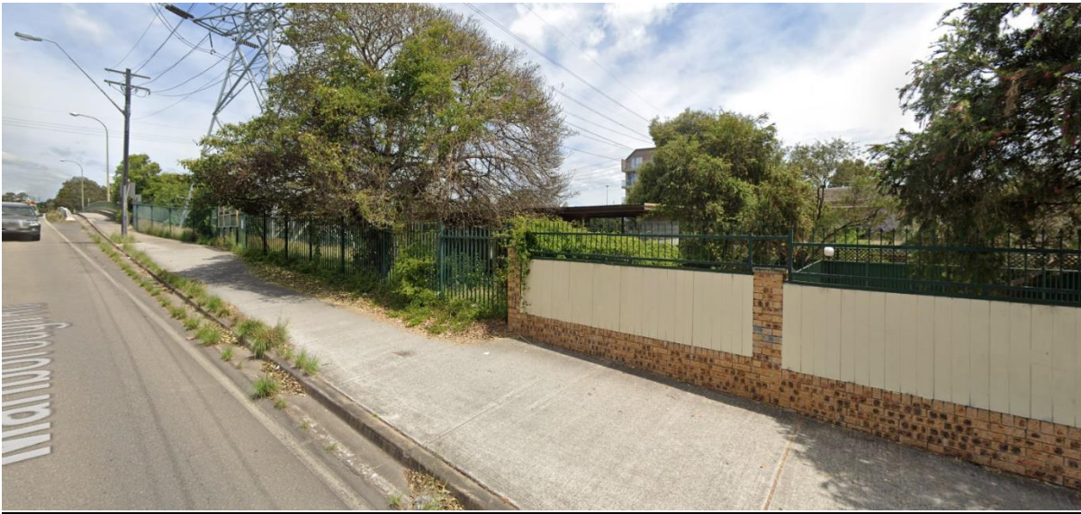
Figure 16 – Street view along Marlborough Road with the pool area of the development at 66-72 Marlborough Road on the right of the photo
