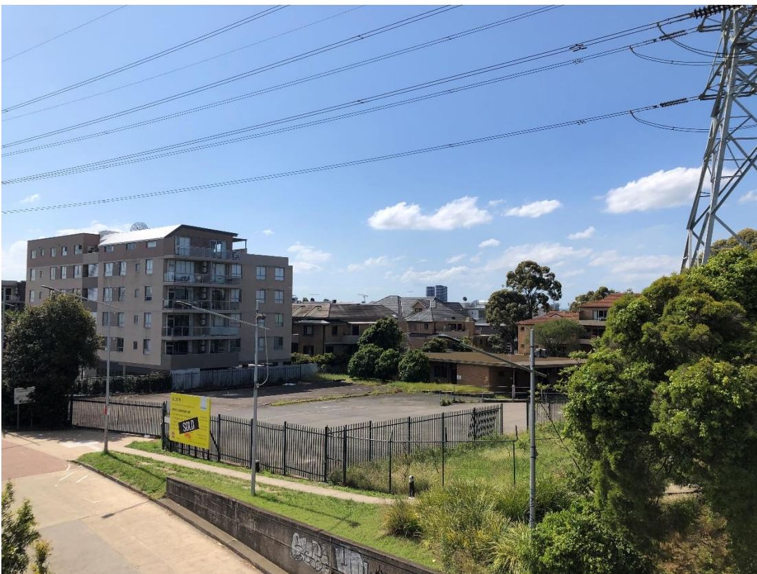
Figure 5 – The subject site as viewed from the Marlborough Road overpass
