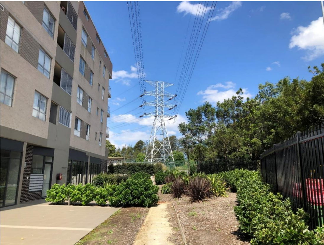
Figure 15 – Looking east towards the site across the front setback of the adjoining development at 81-86 Courallie Avenue
