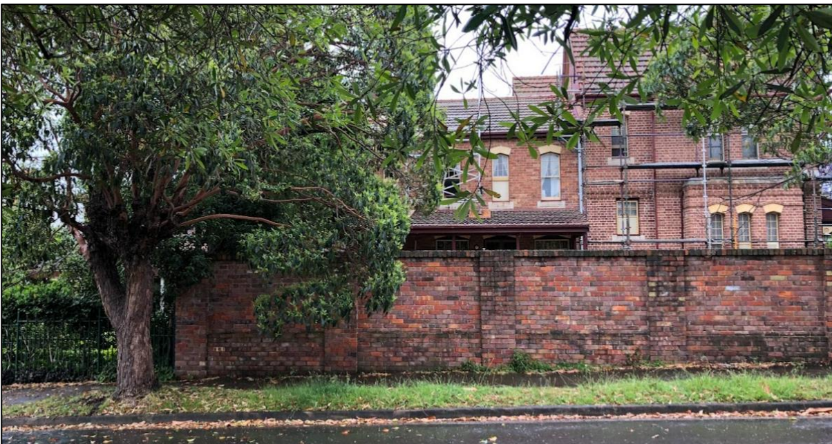
Figure 12: View across the street facing North.
