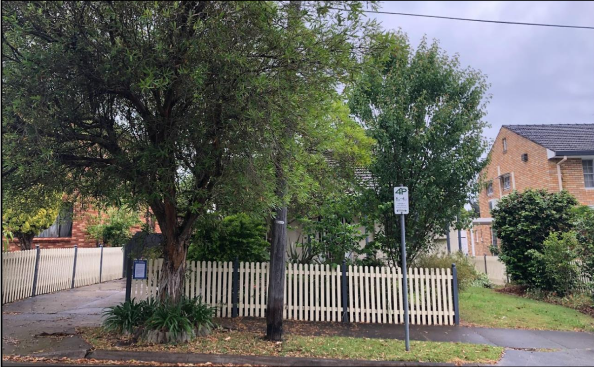
Figure 9: Front view of 12 Alviston Street.
