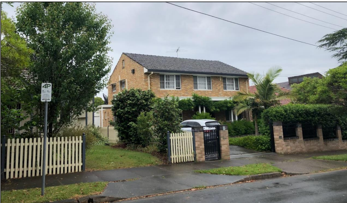
Figure 10: View of western-adjointing neighbouring property at 14 Alviston Street.
