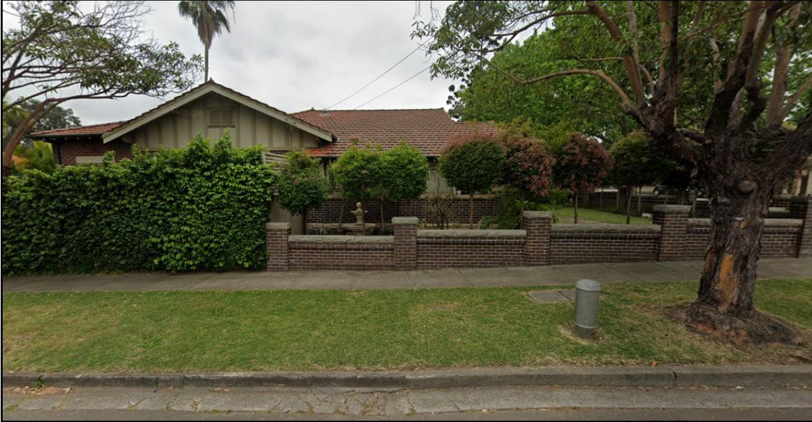
Figure 15: Item 162 – Kiameron Californian bungalow Gelling Avenue frontage
