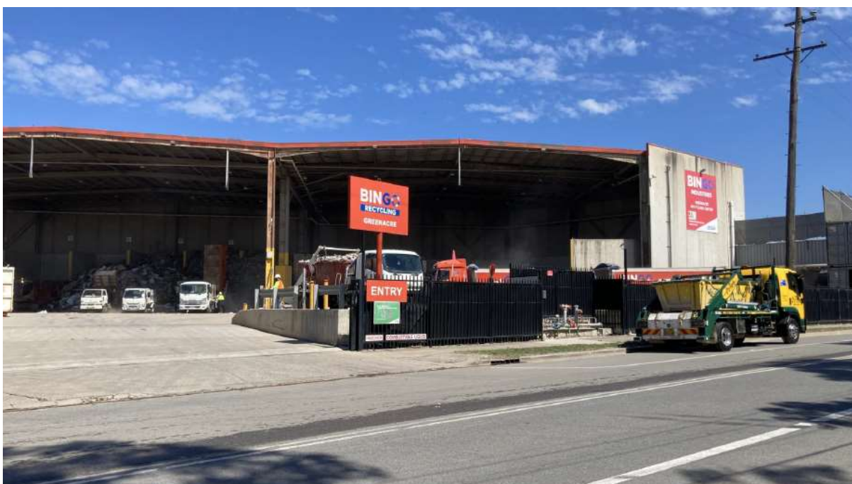
Figure 4. Frontage of the subject site.
