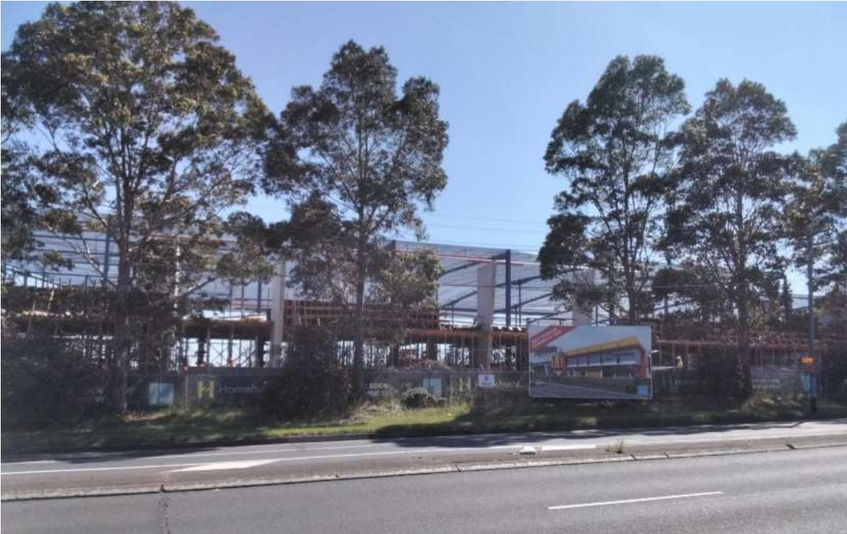
Figure 3. Part of the southern elevation of Building 1 fronting Parramatta Road.
