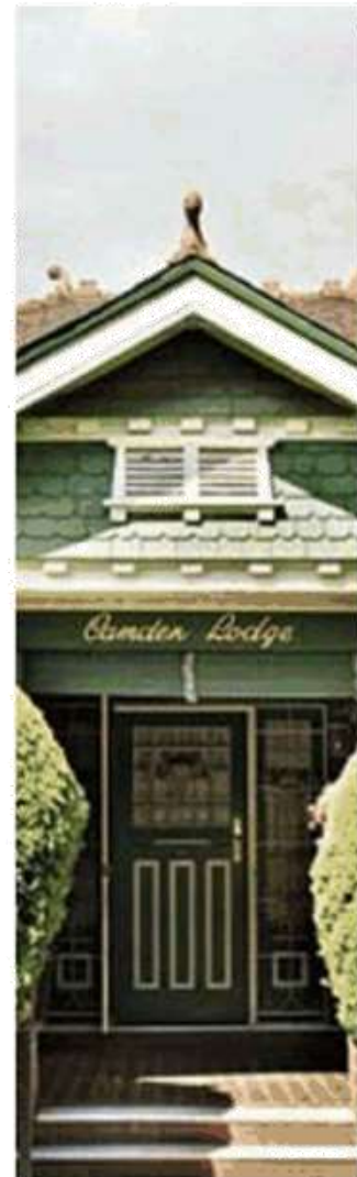
RESTORE CAMDEN LODGE TO ORIGINAL HERITAGE FINISHES
