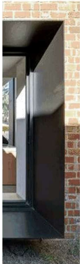
STEEL WINDOW BOX / RECYCLED HERITAGE BRICK
