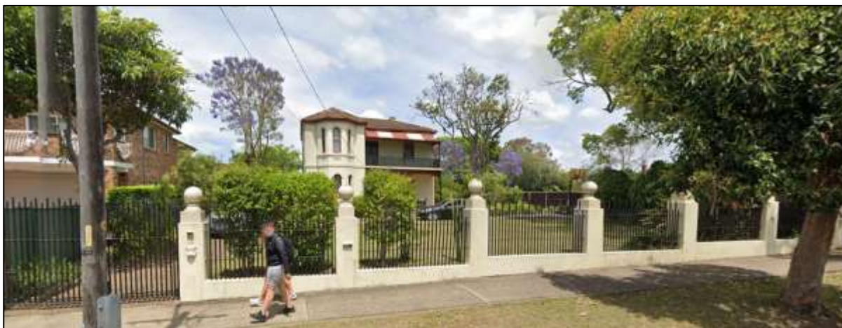
Figure 18: Eastern adjoining Victorian Italianate heritage item (94-96 Burlington Road, Homebush).
