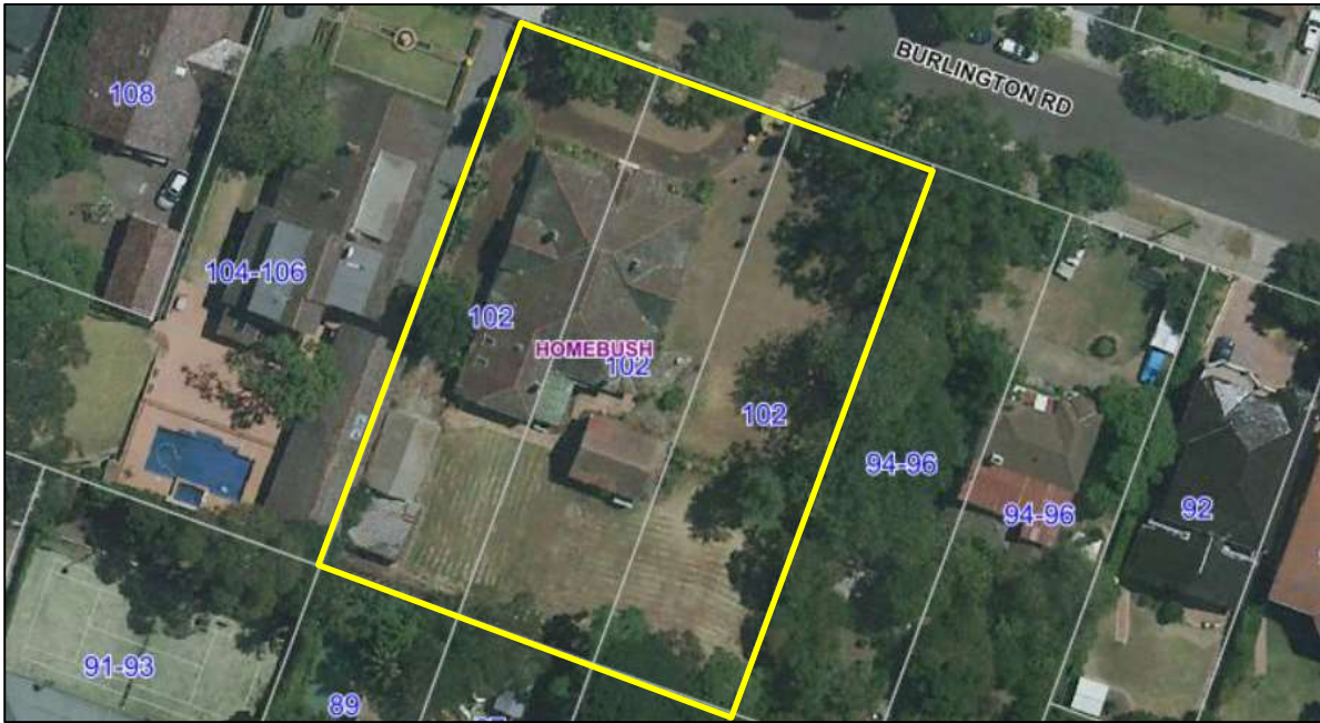
Figure 8: Aerial view of subject site outlined in yellow taken in 2011 before fire damage.
