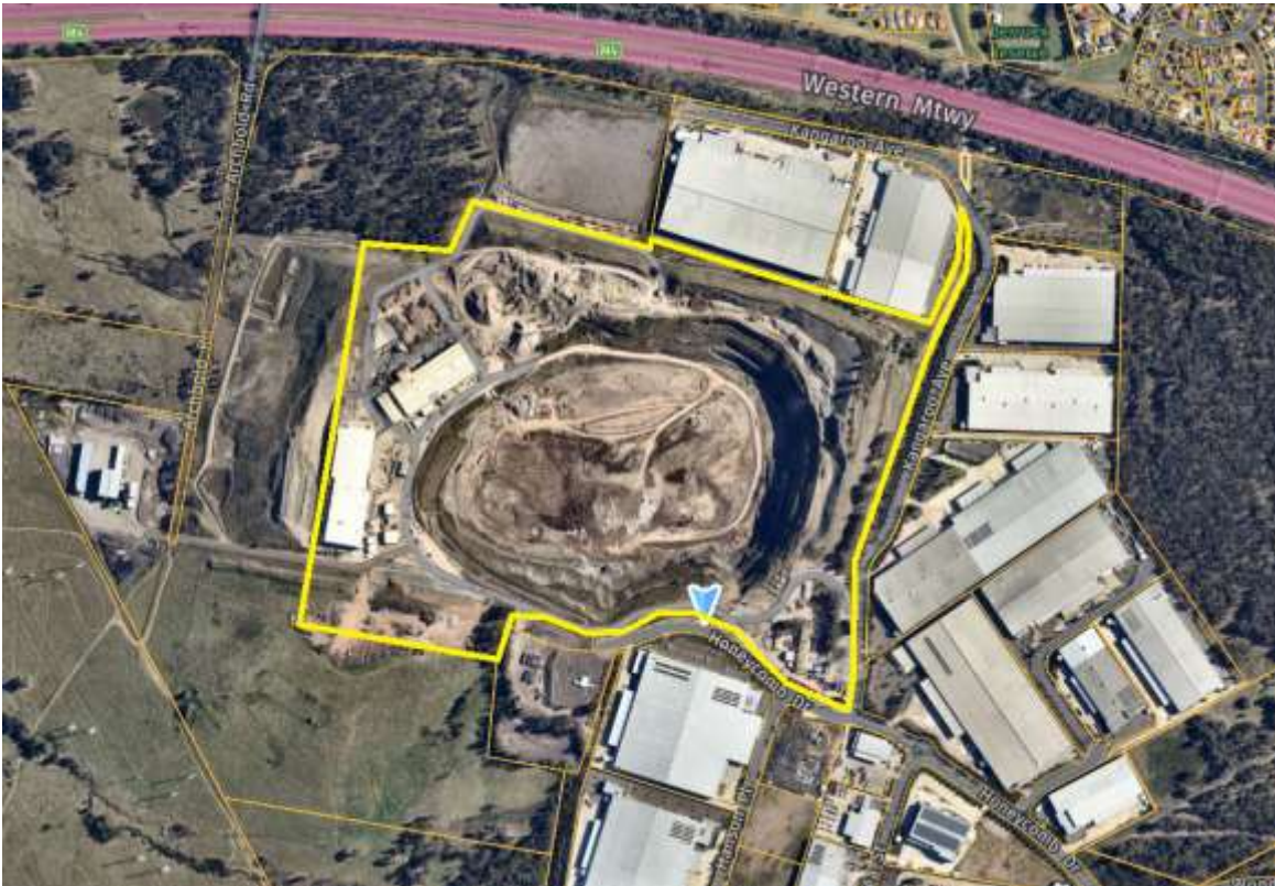
Figure 8. Bingo Eastern Creek Recycling Facility (outlined) and the immediate locality.
