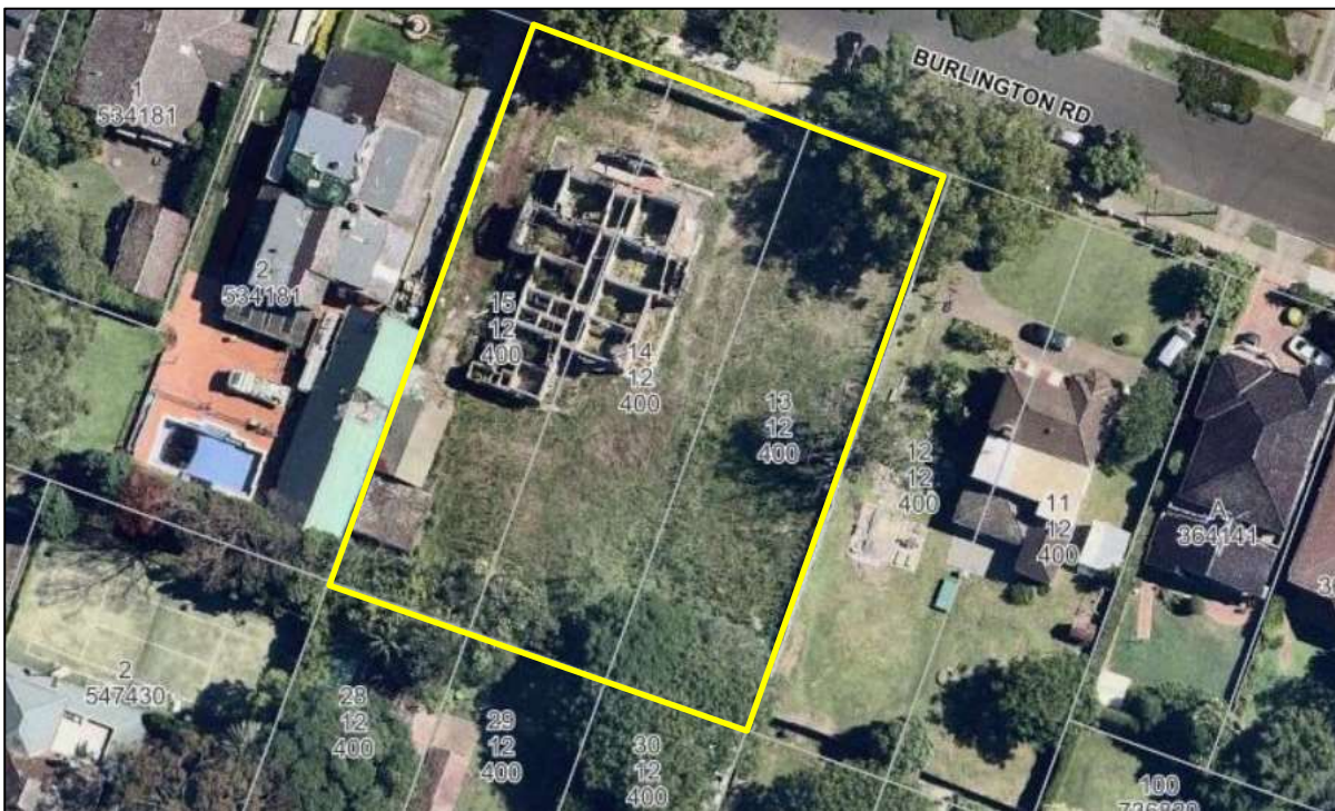
Figure 9: Aerial photo of subject site outlined in yellow in its current state noting severely dilapidated state of the dwelling.
