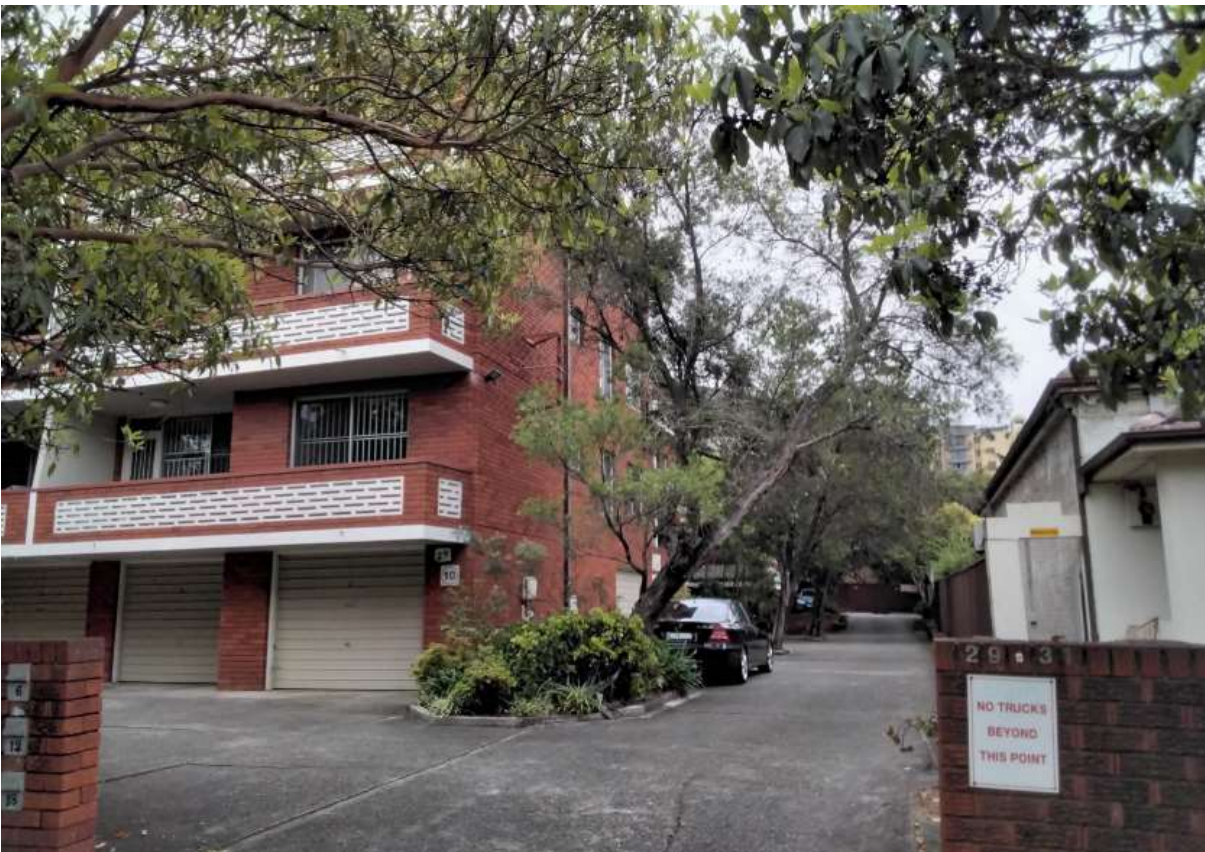
Figure 21. Four-storey residential flat building - 29-31 Albert Rd.
