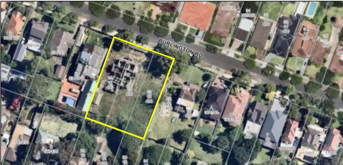
Figure 1: Aerial view of subject site outlined in yellow and surrounding context.
