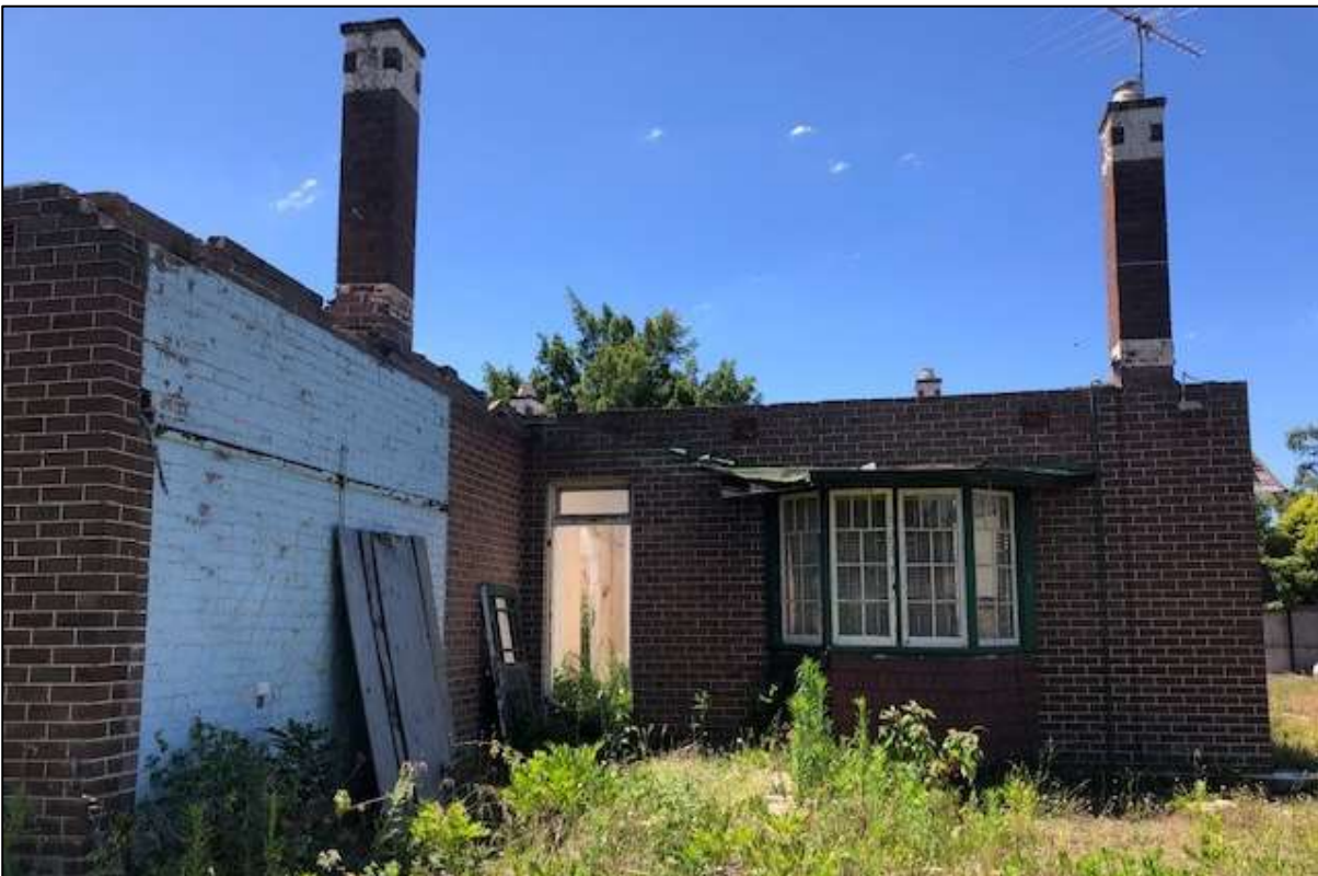
Figure 13: Rear southern elevation of the dwelling proposed for demolition.
