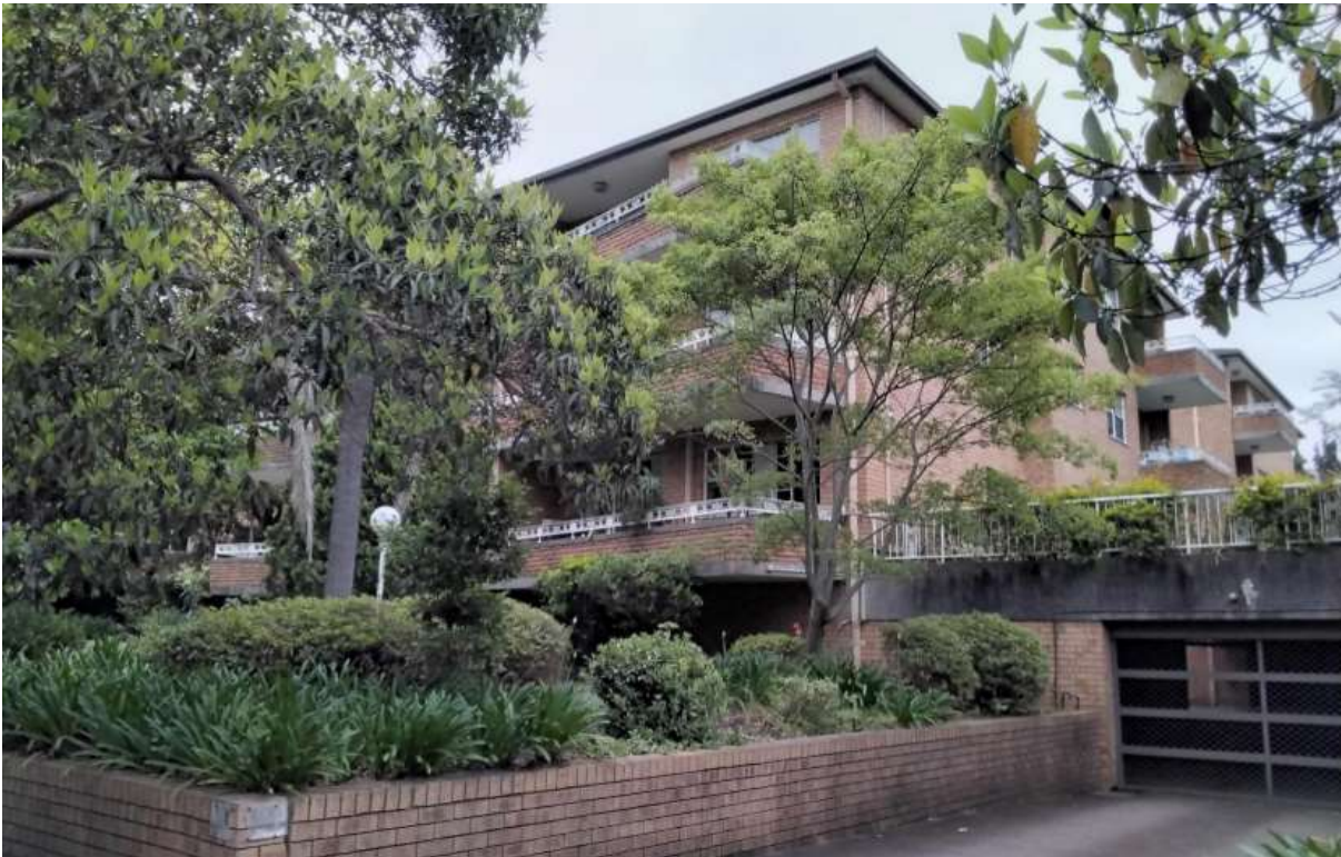
Figure 22. Three to four-storey residential flat building – 33-39 Albert Rd.
