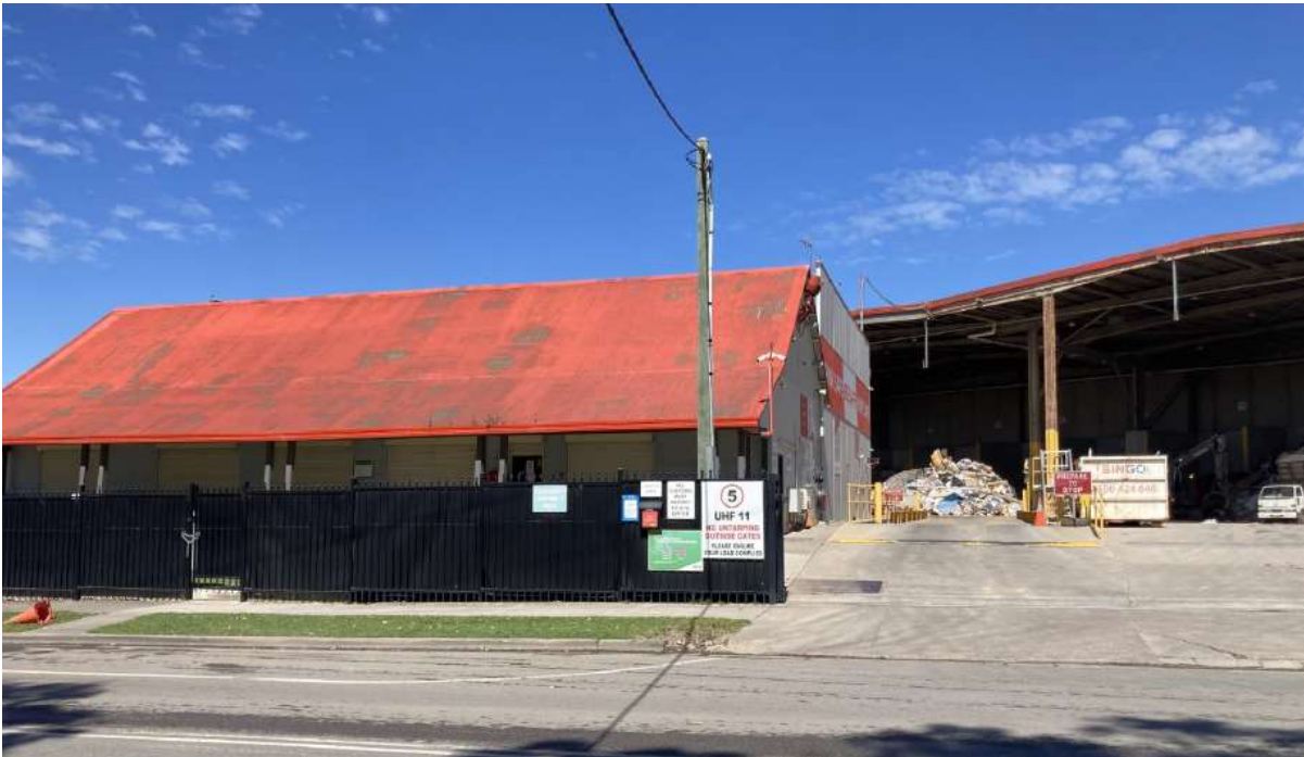
Figure 5. Frontage of the subject site.
