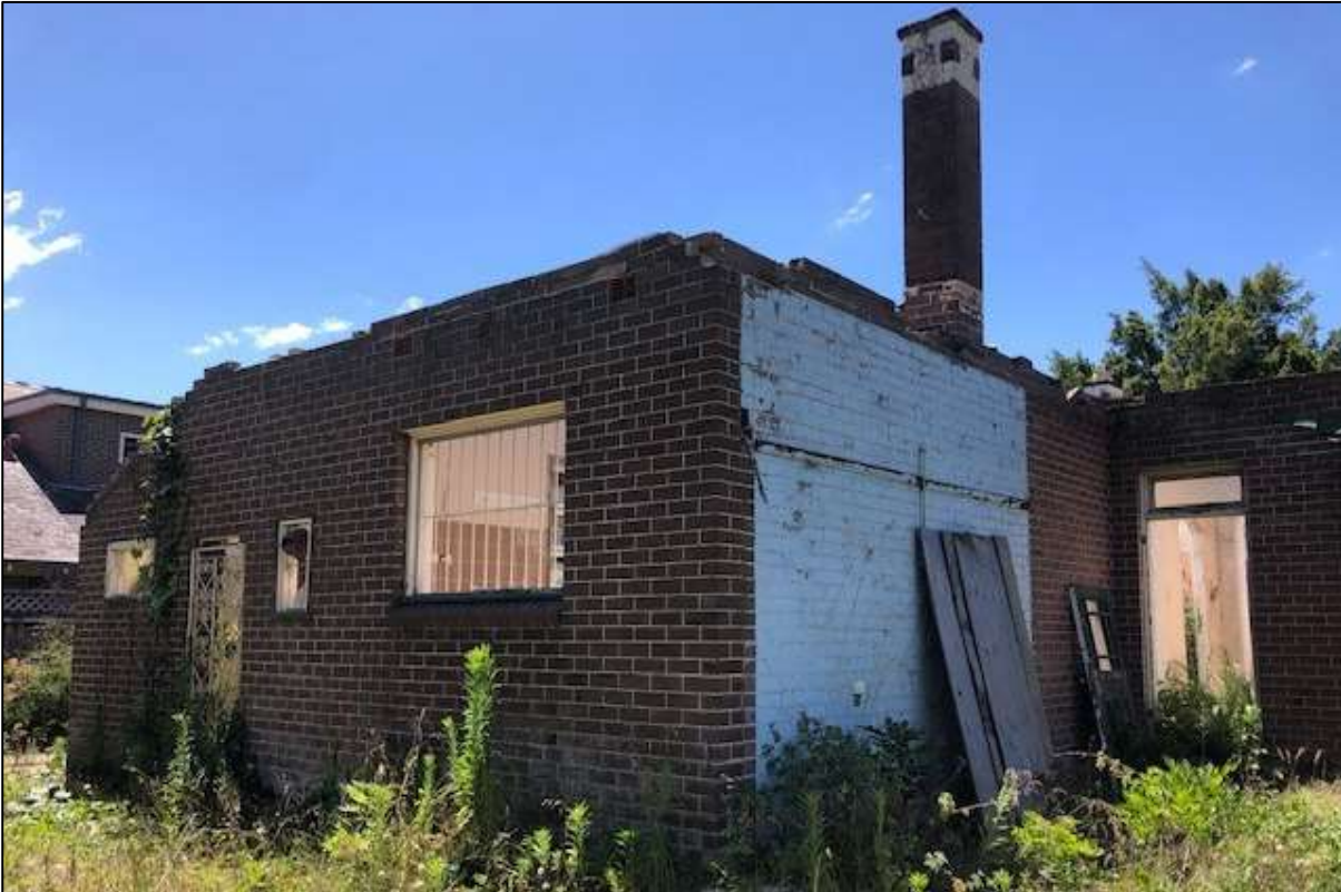
Figure 12: Rear southern elevation of the dwelling proposed for demolition.
