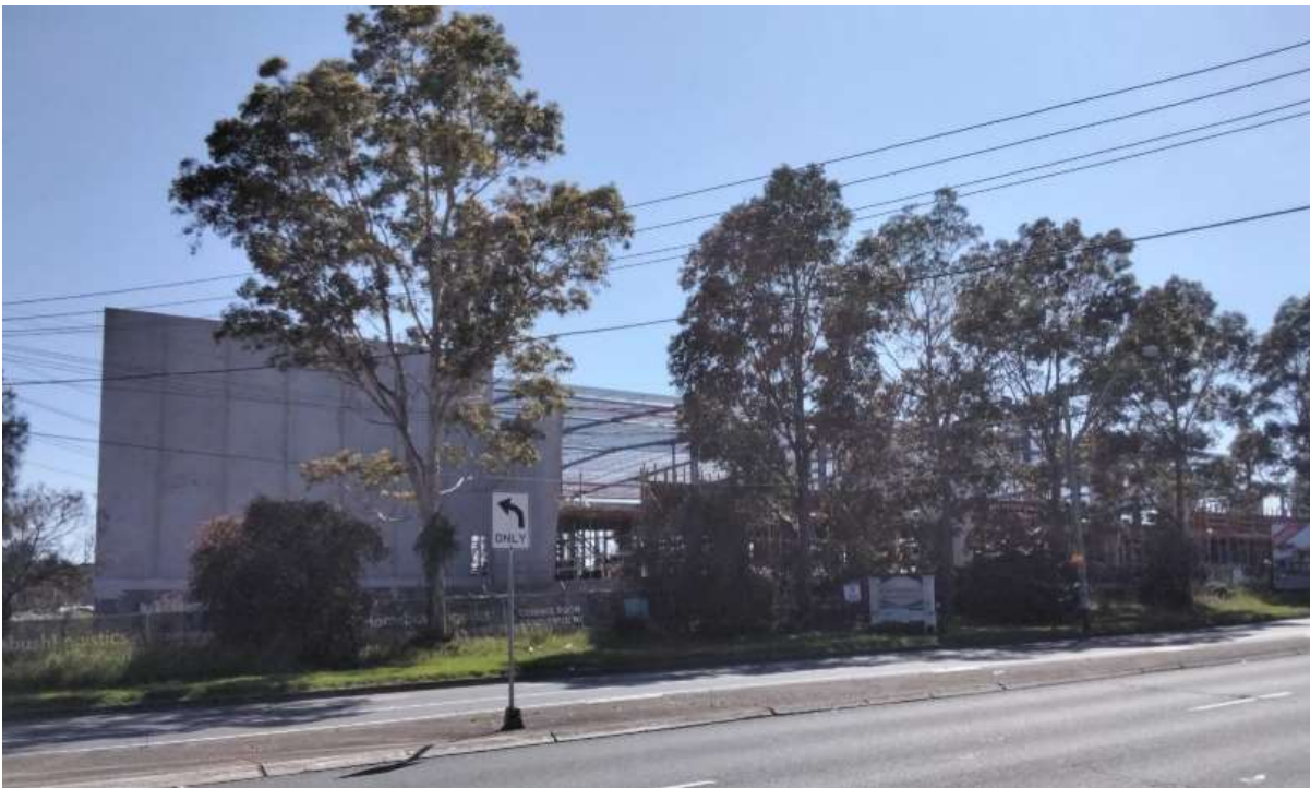
Figure 2. Southern elevation of Building 1 (fronting Parramatta Road).
