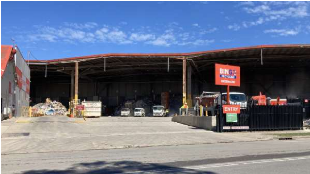
Figure 7. Front of the existing recycling facility on the subject site.
