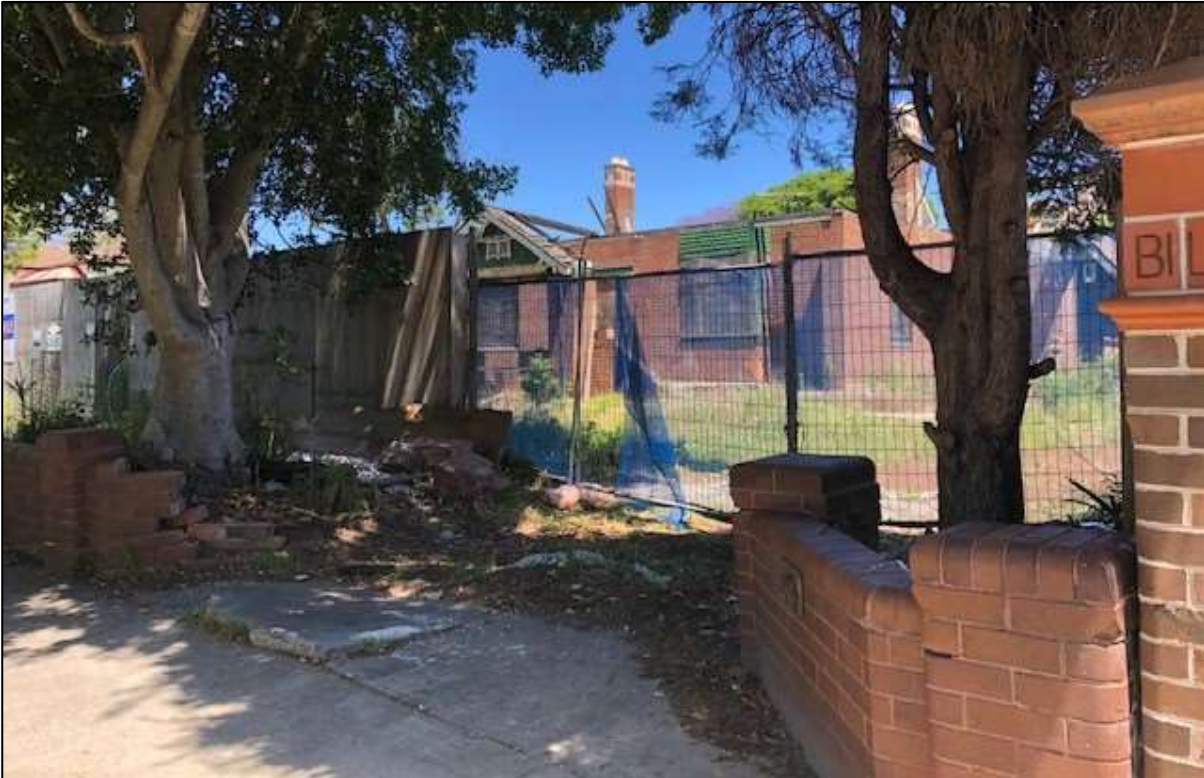
Figure 16: North-western driveway entrance showing dilapidated fencing. Both trees either side of the driveway are proposed for removal.
