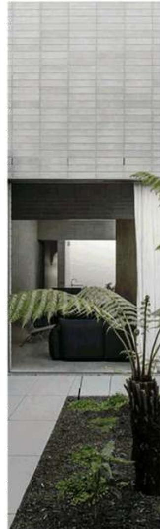
EXPOSED BRICK FINISH
