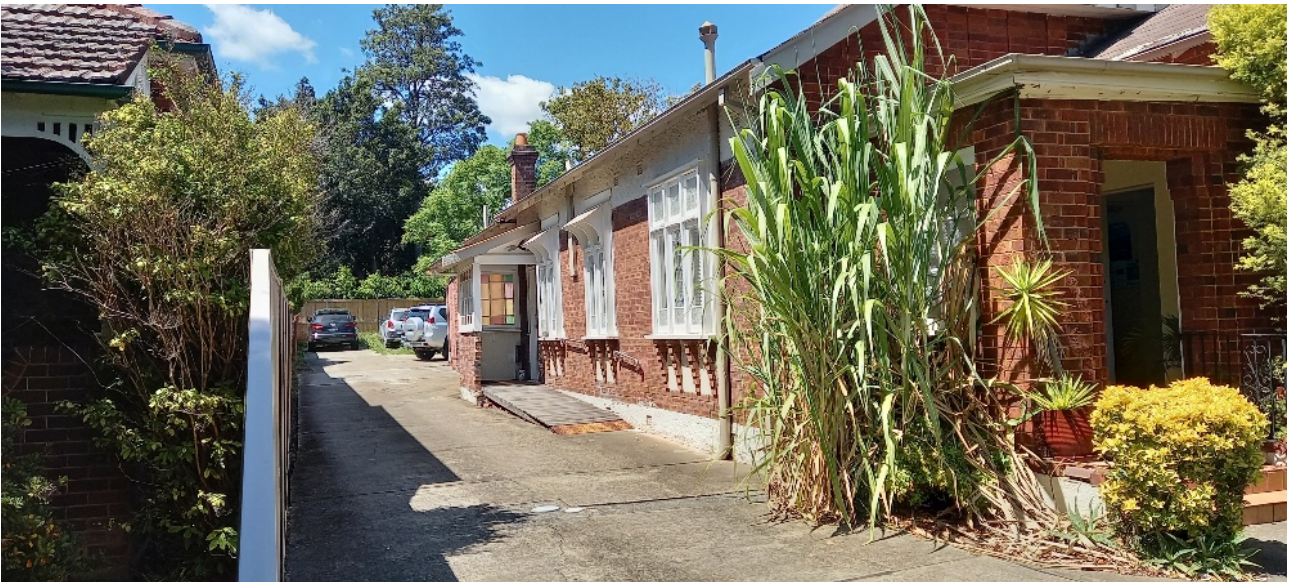
Figure 7. Northern elevation of adjoining dental surgery to the south (16 Rochester Street) on R2 low-density residential zoned land. At-grade car parking to the surgery is located at the rear.
